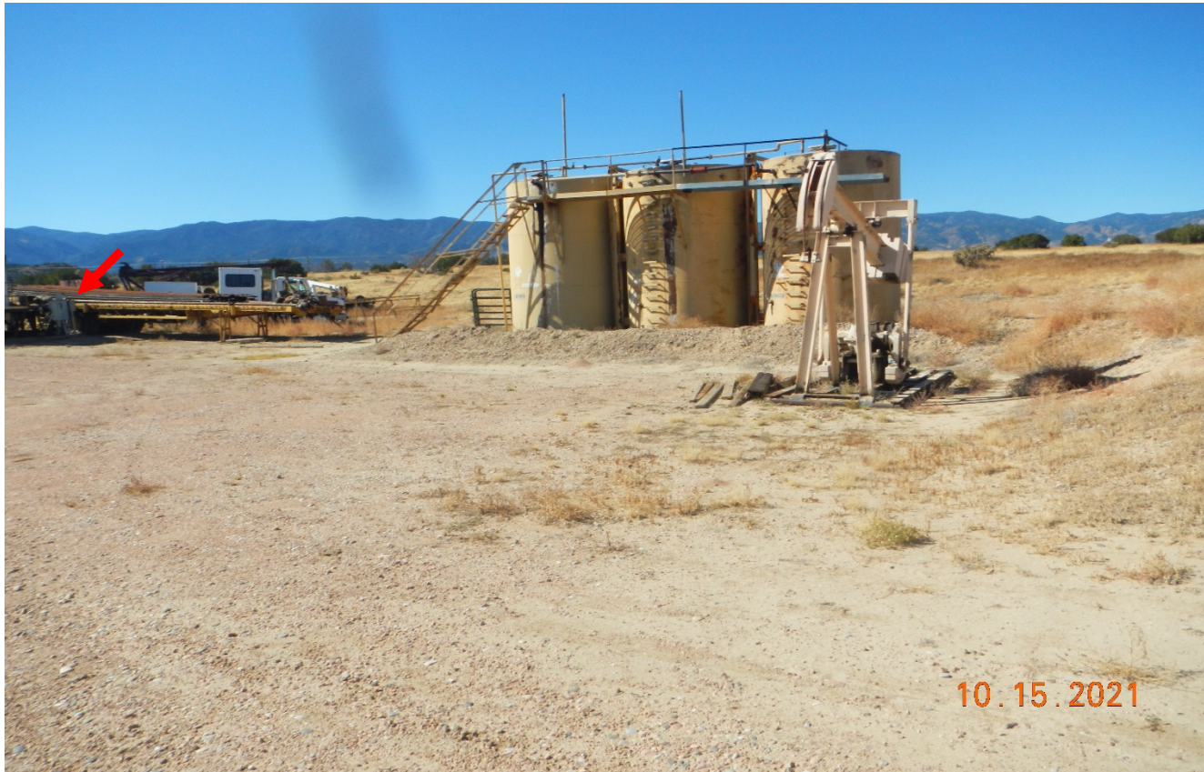
Photo 3. Facing west at the well site. The pumpjack has been disconnected from the well. The well is shown at red arrow. The well appears to be temporarily abandoned.
