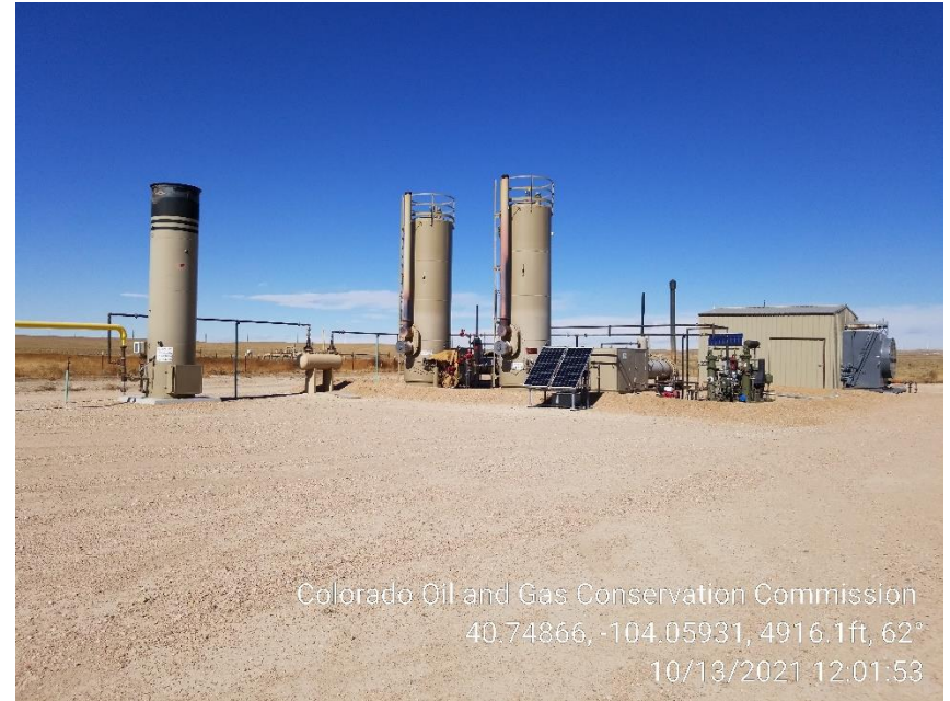
Photo 6 – Separators and ECD
