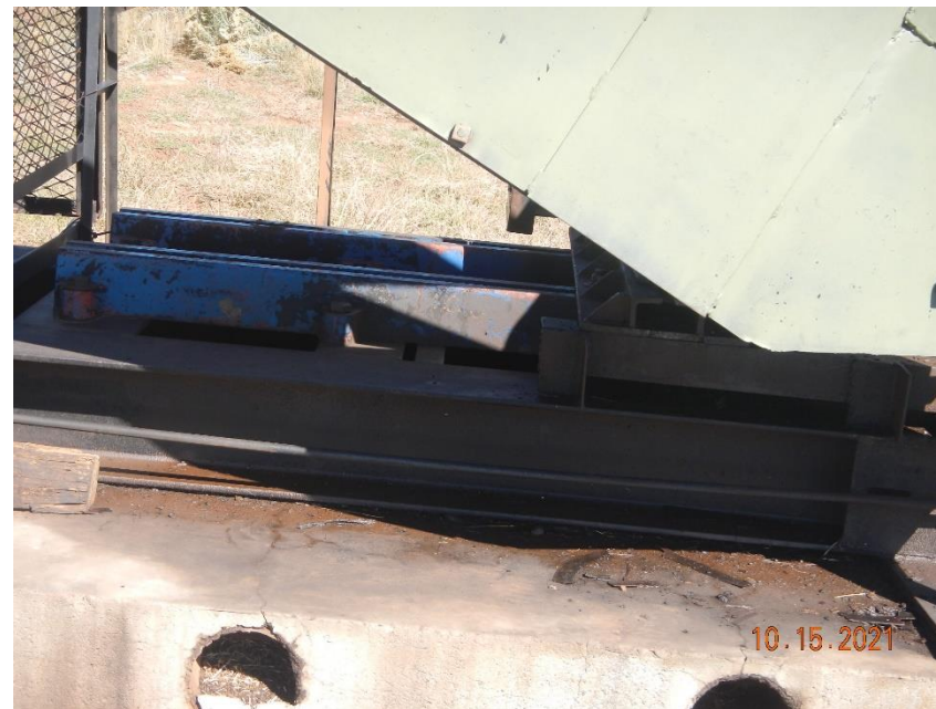
Lube oil accumulating
