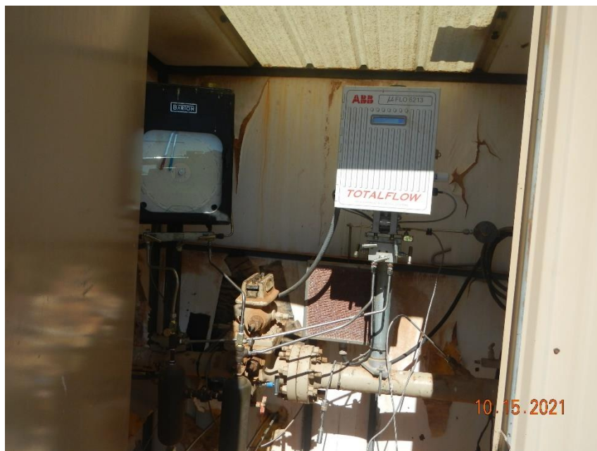
No gas meter calibration record visible
