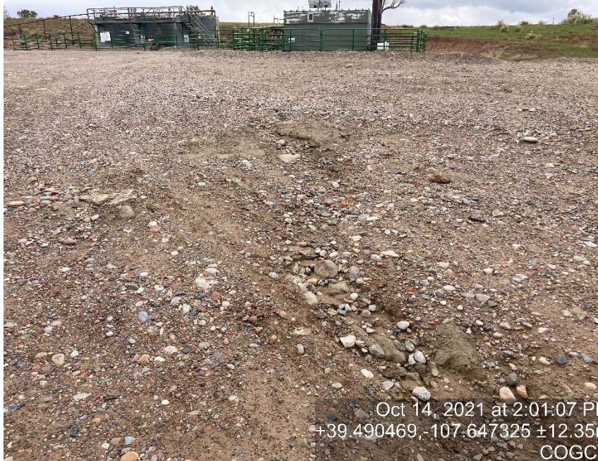
Lack of stabilization/erosion
