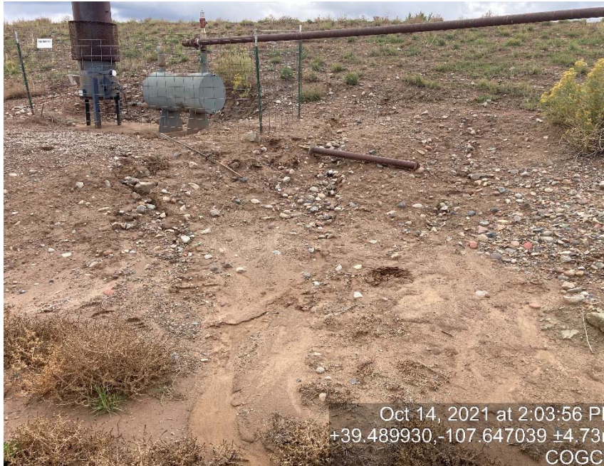
Lack of stabilization/erosion
