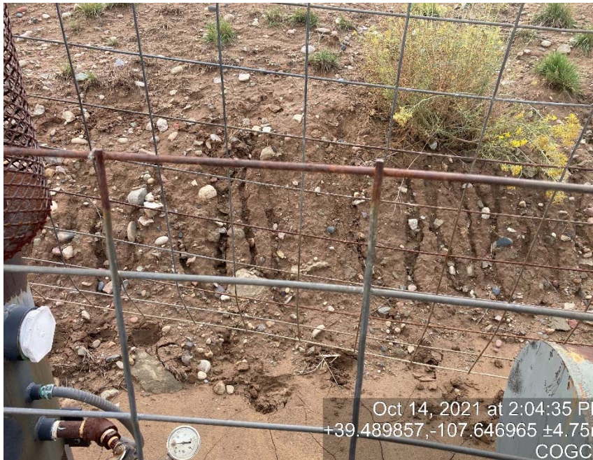
Lack of stabilization/erosion
