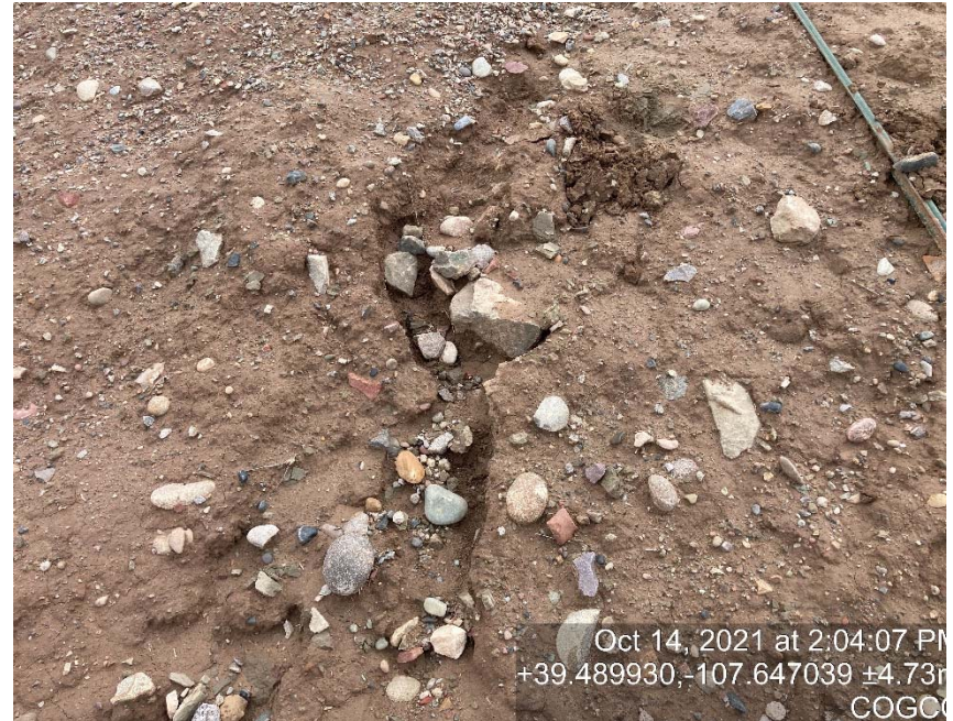
Lack of stabilization/erosion
