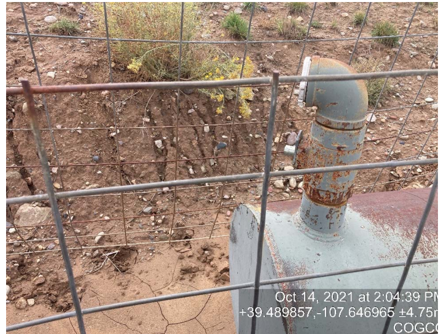
Lack of stabilization/erosion
