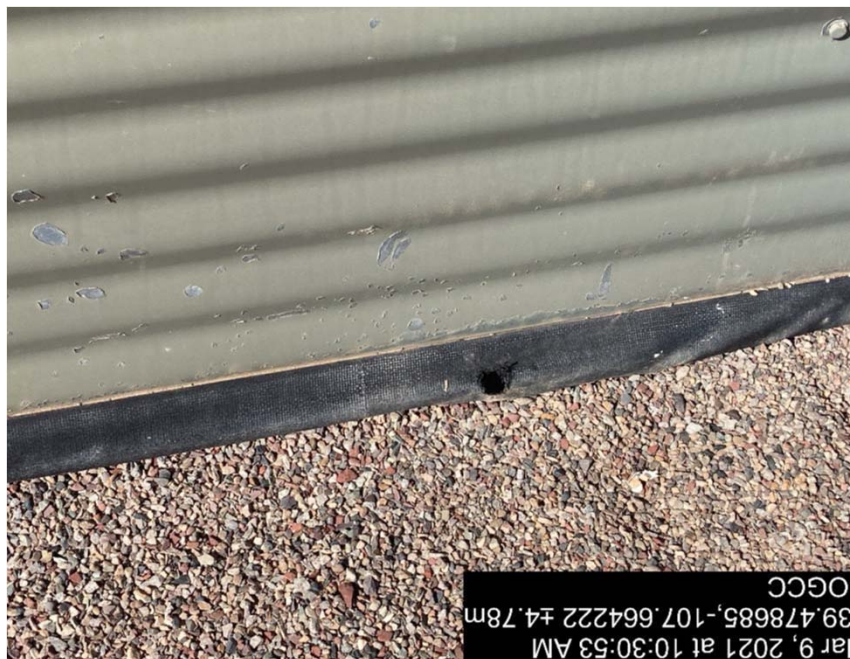
Previous inspection photo
