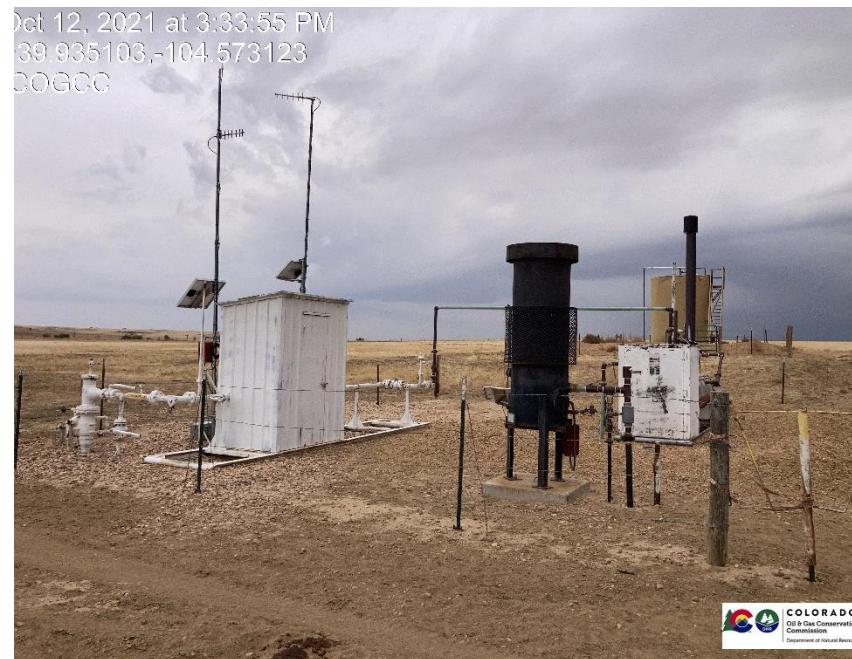
Pic 2 separator, gas meter run, ECD
