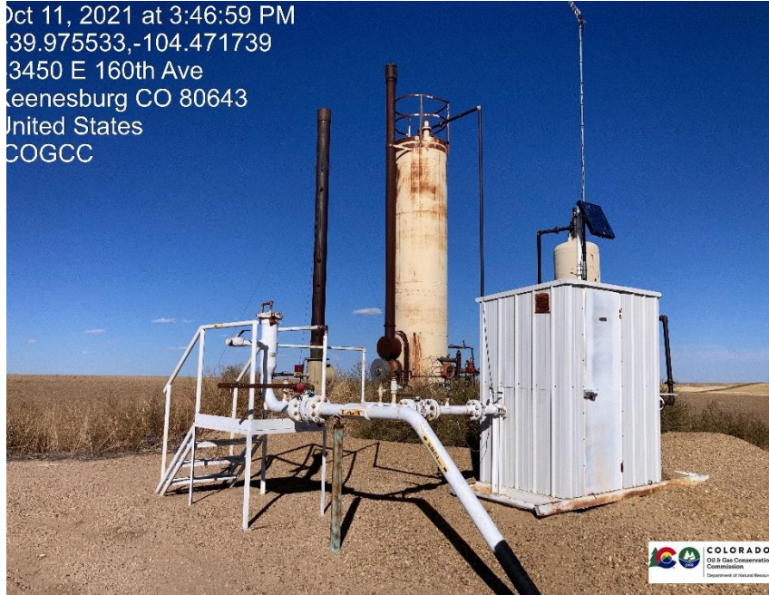
Pic 3 gas meter run, vertical separator, ECD
