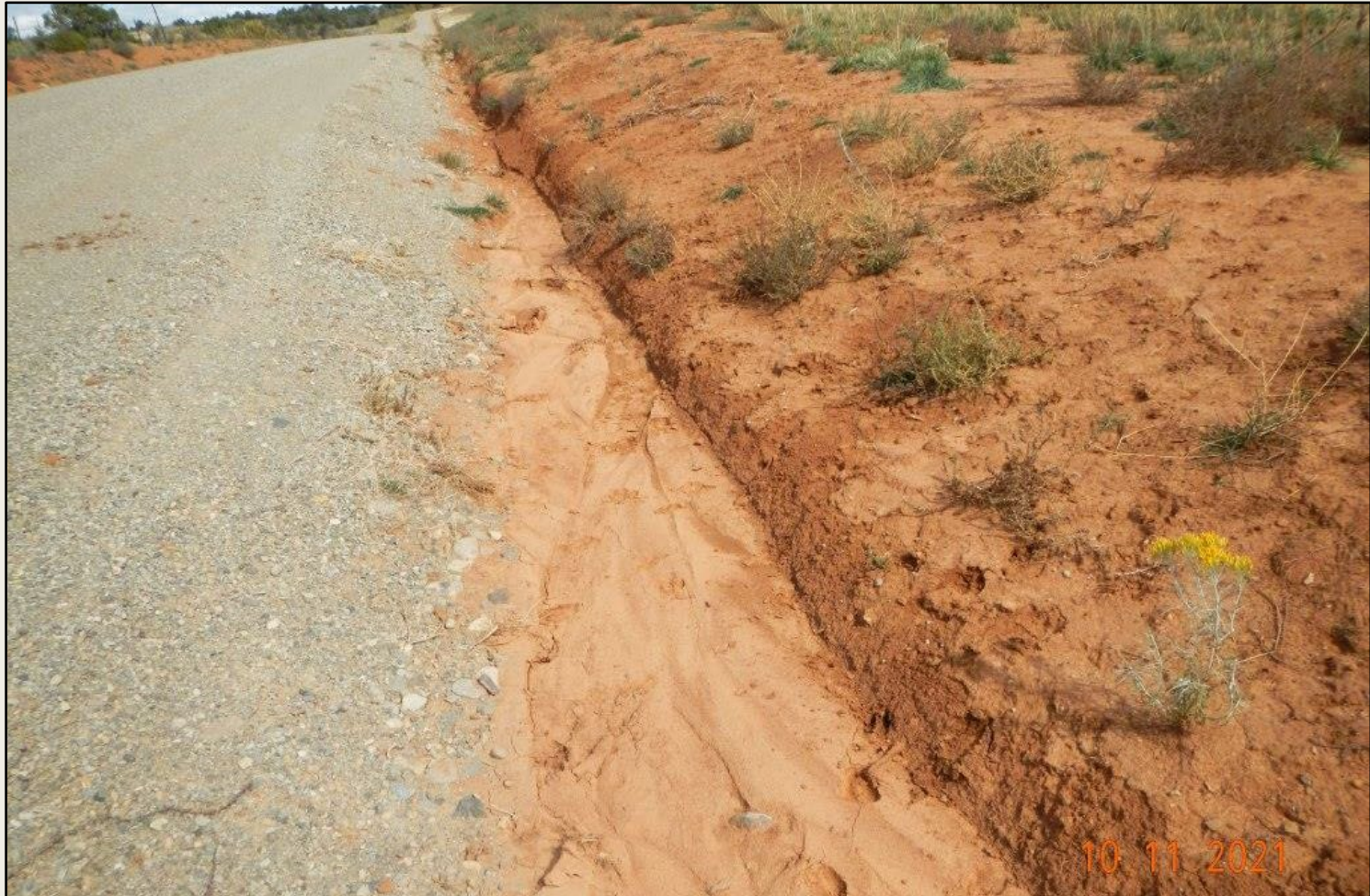
Photo 7. View of area along the access road where volumes of sediment are eroding down-slope. Additional stormwater and erosion control BMPs are needed here.
