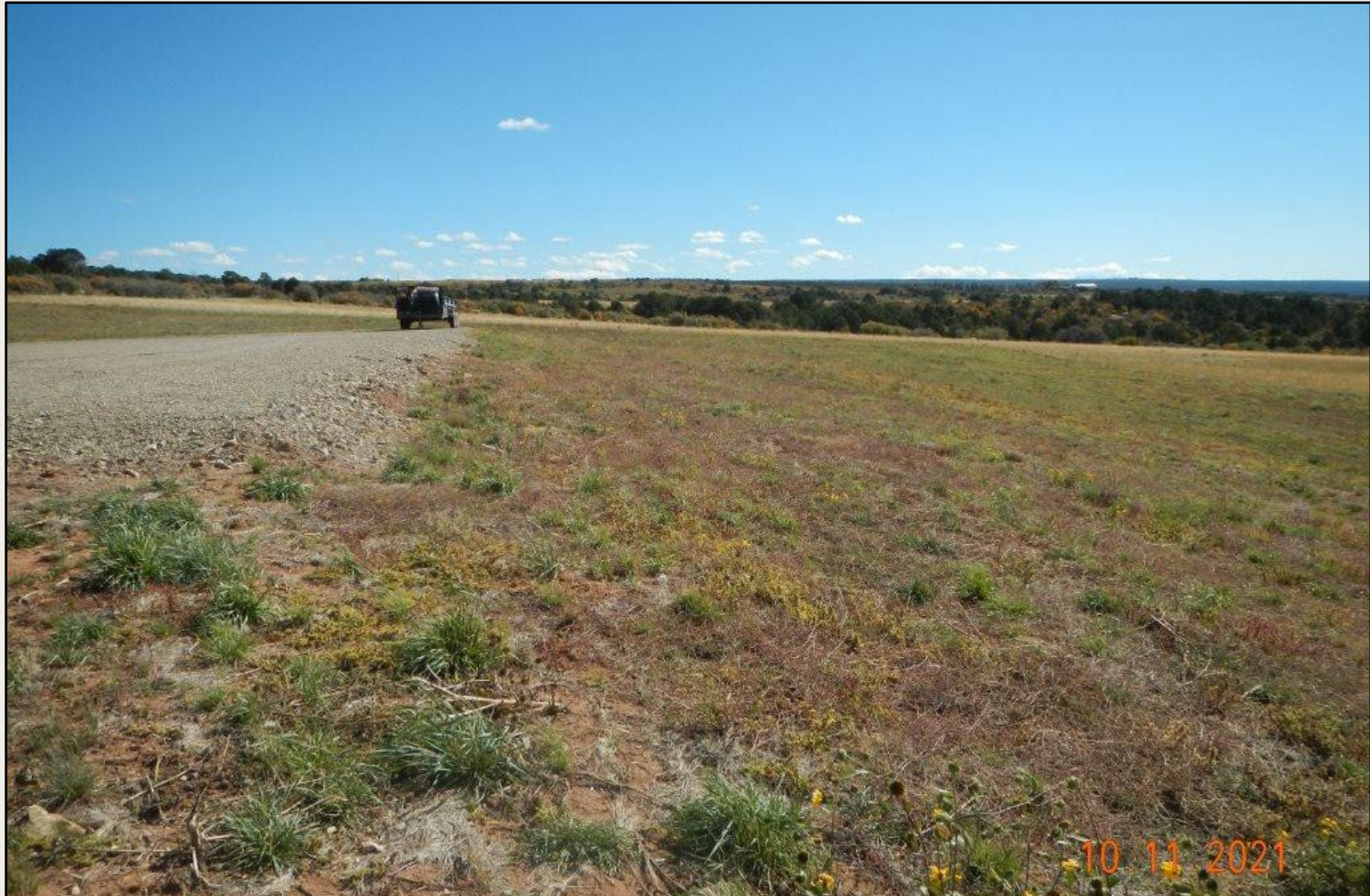
Photo 2. View of the southern fill slope from the southwestern corner facing eastward. Revegetation is progressing with grasses in an early identifiable condition that appears to be intermediate wheatgrass, blue grama, western wheatgrass, as well as forbs such as showy goldeneye, penstemon, and purple asters.
