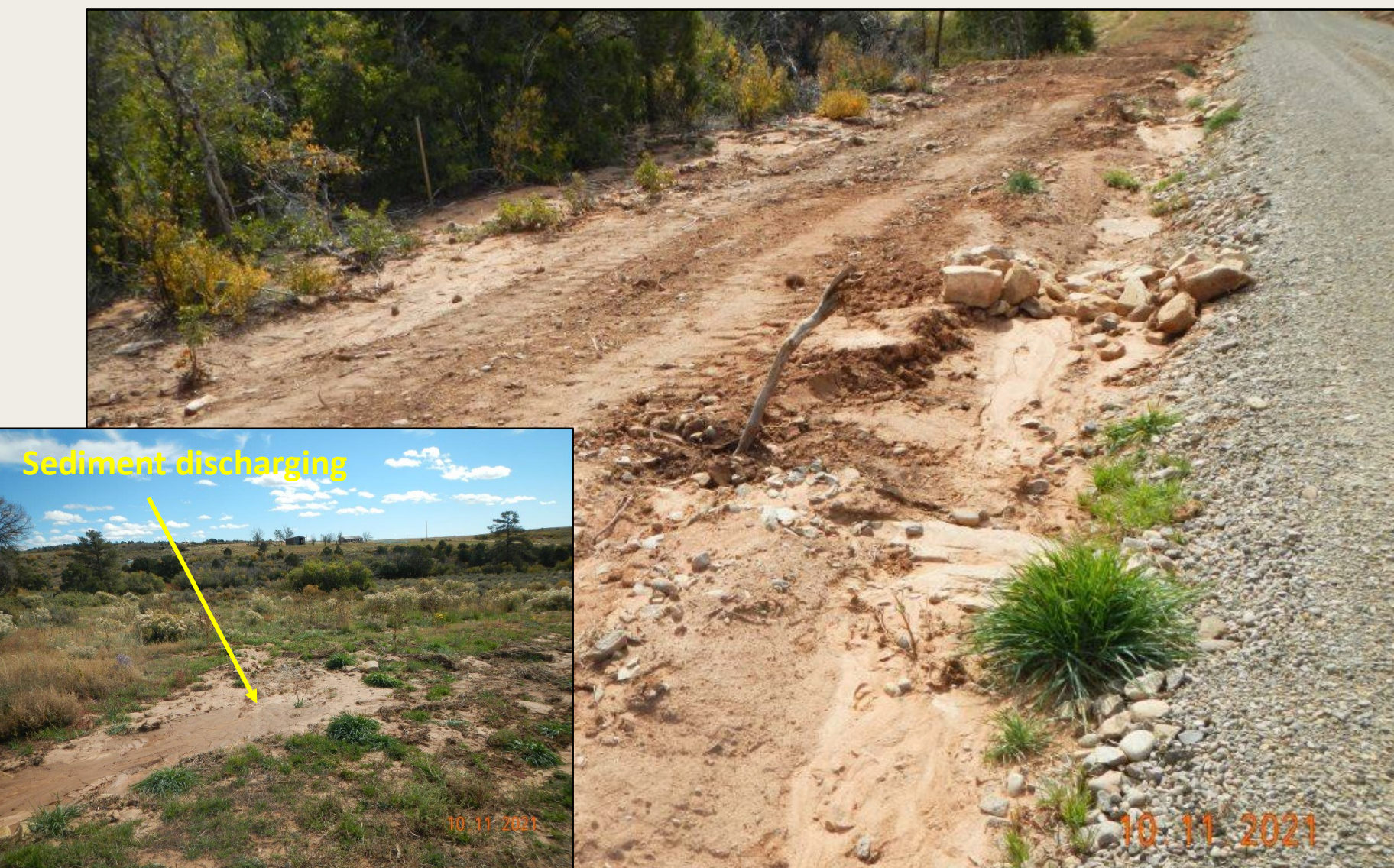
Photo 8. View of another area along the access road with evidence of sediment transport, and where existing BMPs are not adequate. Graded area adjacent to roadside ditch needs revegetation. Inset shows sediment discharge at bottom of slope.
