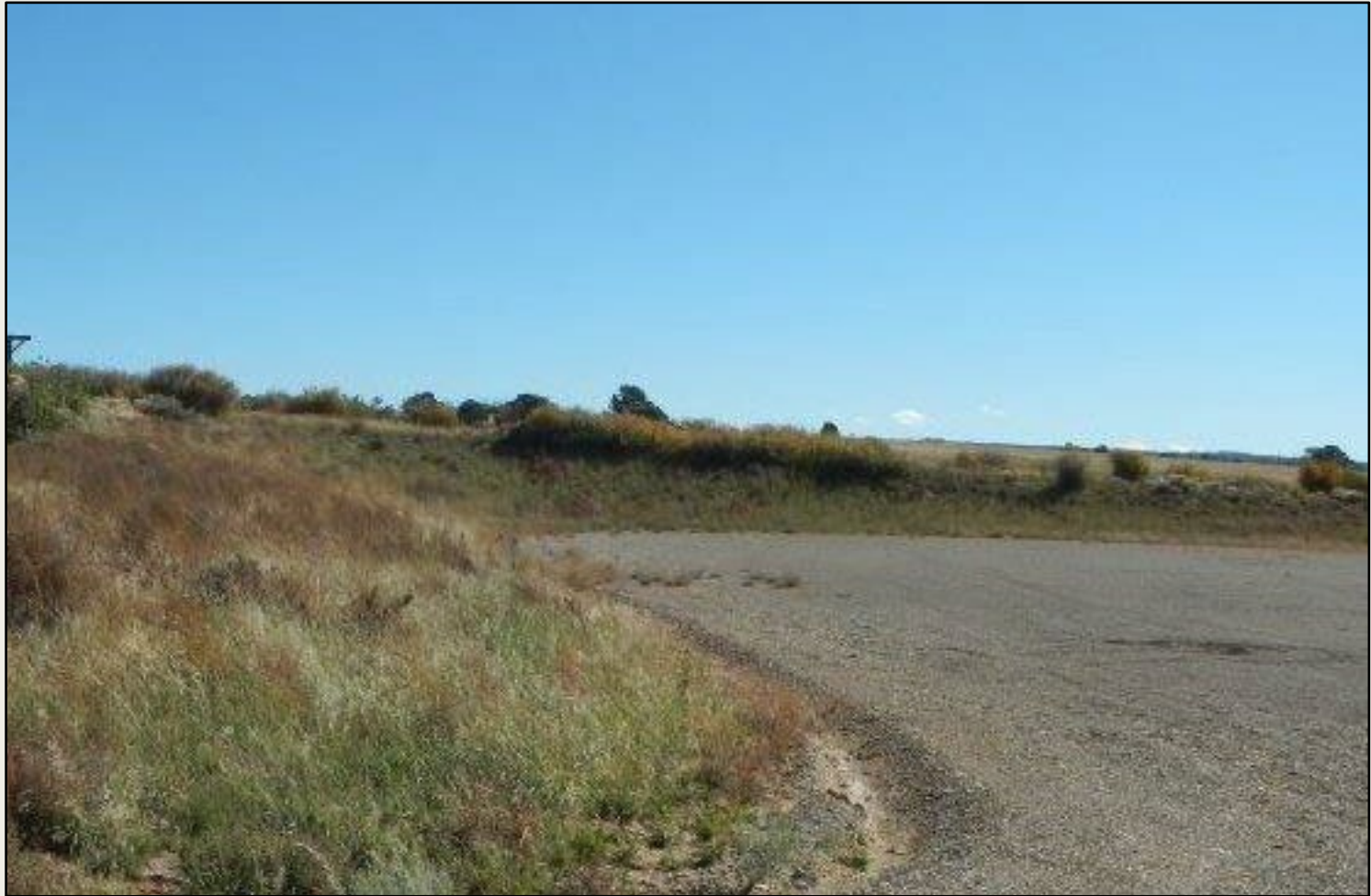
Photo 2. View of well pad cut-slopes. Per conditions of approval on variance. Slopes need to be reduced to a maximum of 3:1. This work is not conducted.
