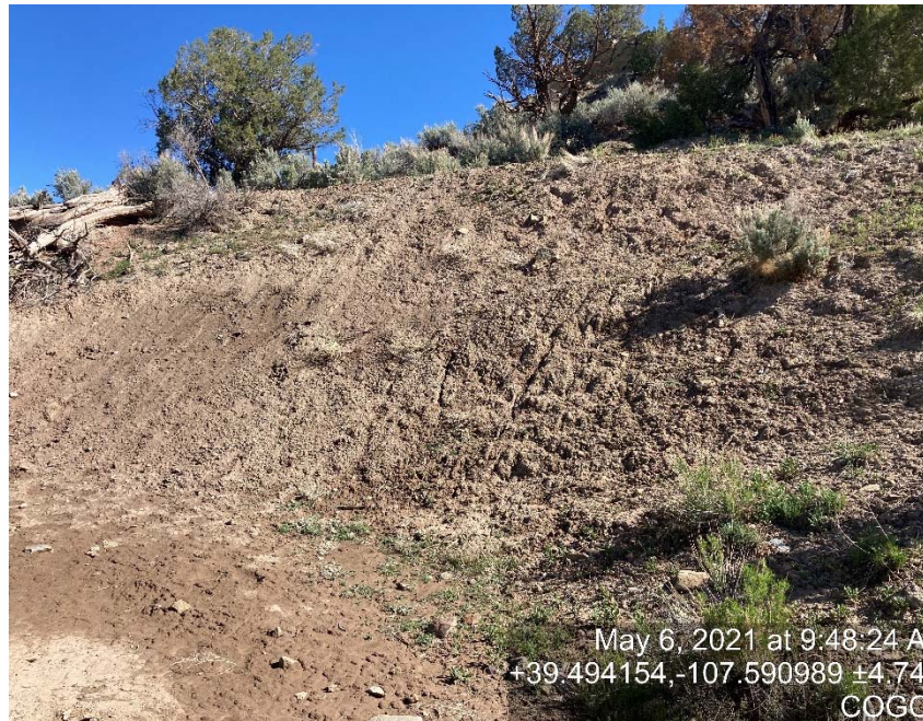
Photo from second inspection document # 700702702 of lack of stabilization/erosion
