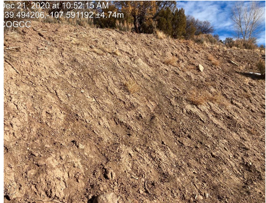
Photo from first inspection document # 700702048 of lack of stabilization/erosion
