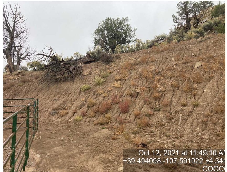
Photo from third/this inspection document # 700703365 of lack of stabilization/erosion
