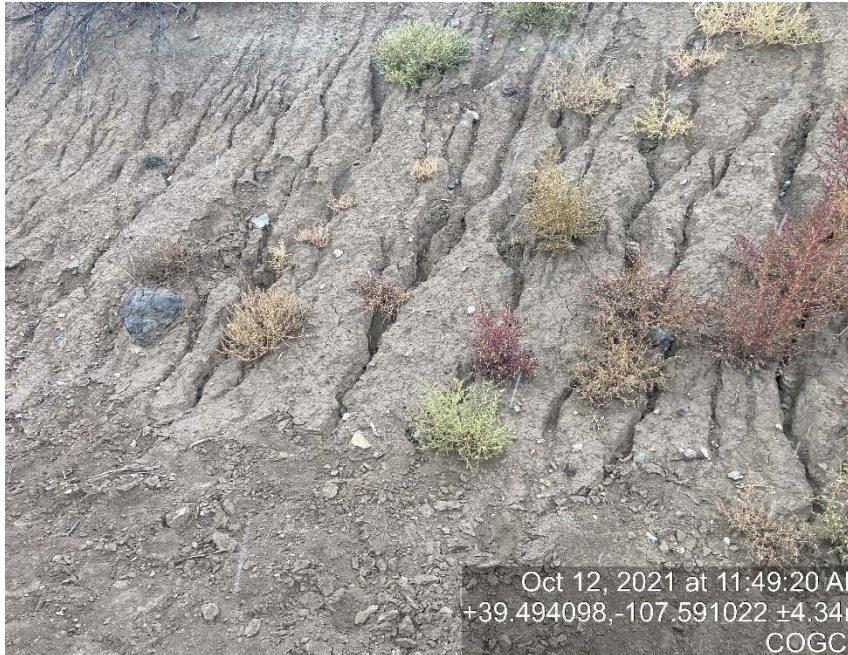
Photo from third/this inspection document # 700703365 of lack of stabilization/erosion
