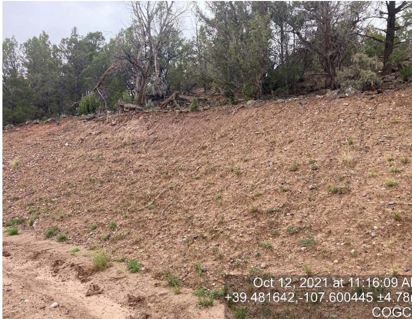
Lack of stabilization/erosion
