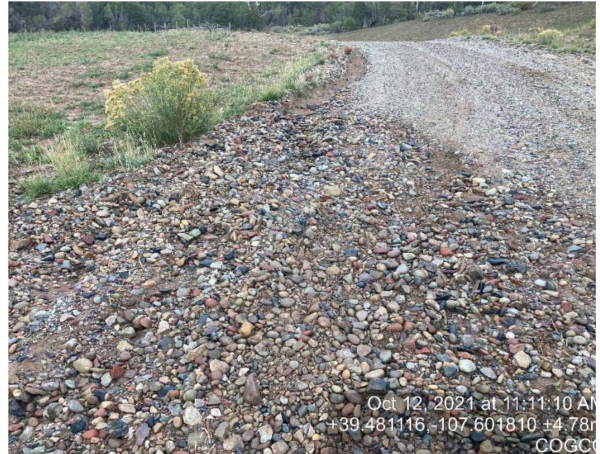
Access road washed out from failing ditch
