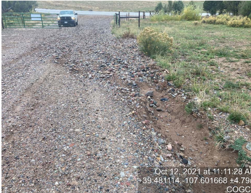
Access road washed out from failing ditch
