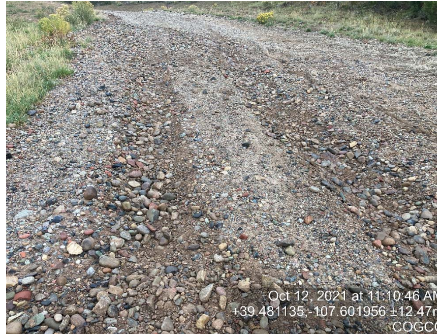
Access road washed out from failing ditch
