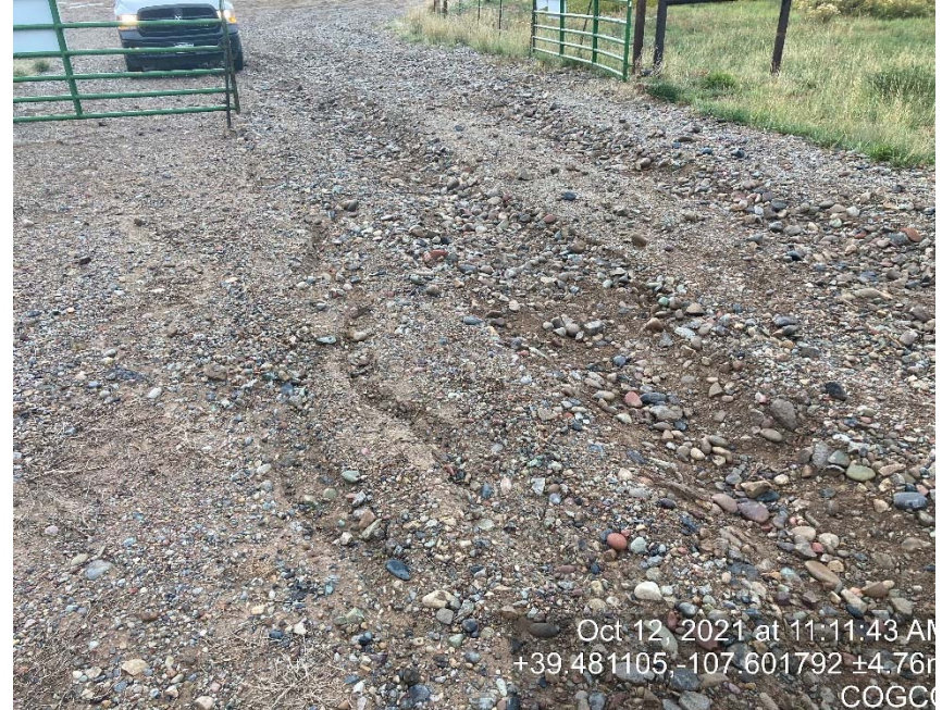
Access road washed out from failing ditch
