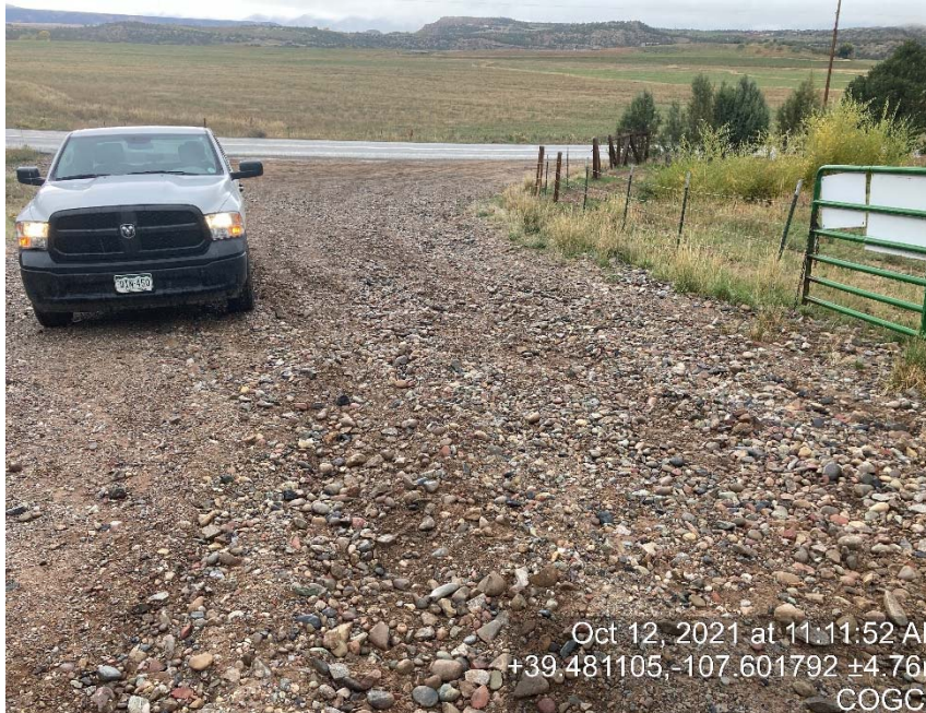
Access road washed out from failing ditch
