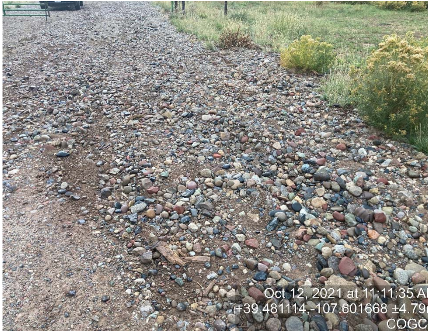
Access road washed out from failing ditch
