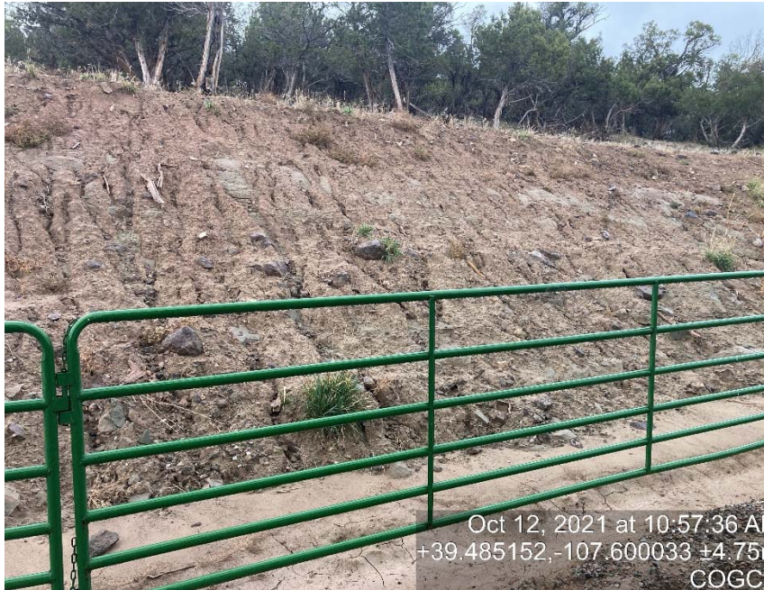
Cut slope lack of stabilization/erosion/riling
