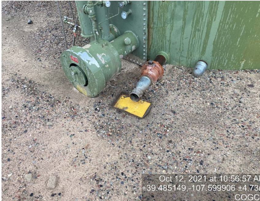
Bull plug/cap missing on load out line
