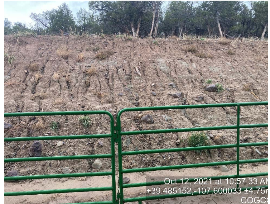
Cut slope lack of stabilization/erosion/riling
