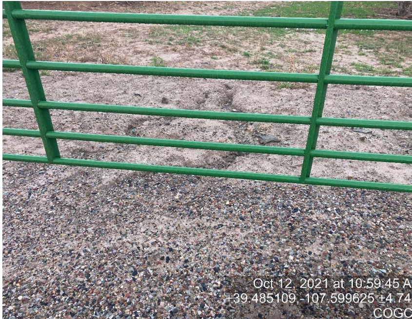
Fill slope erosion/sediment migration
