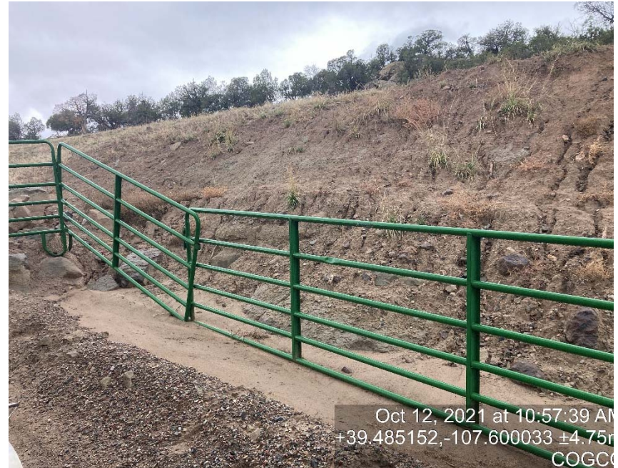
Cut slope lack of stabilization/erosion/riling
