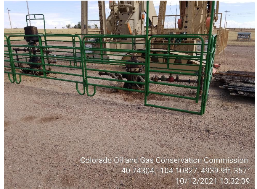
Photo 2 – 1-20-9-60 Wellhead – Stained Soil
