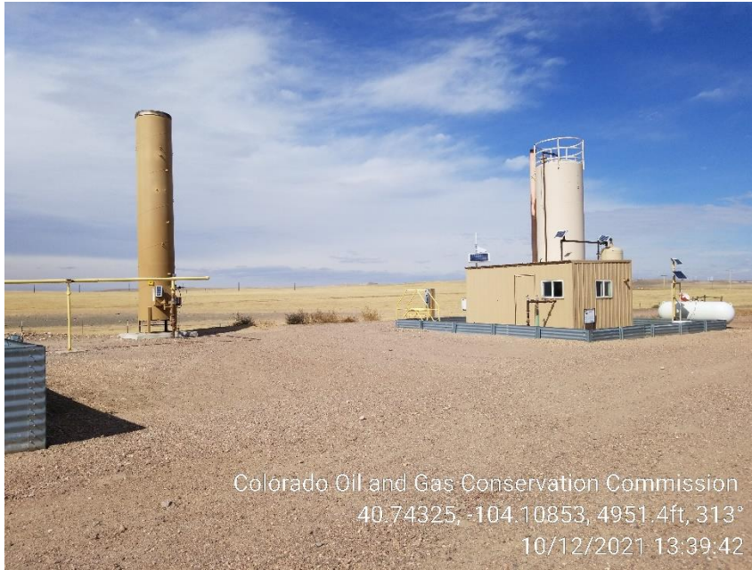
Photo 7 – Heater Treater and ECD
