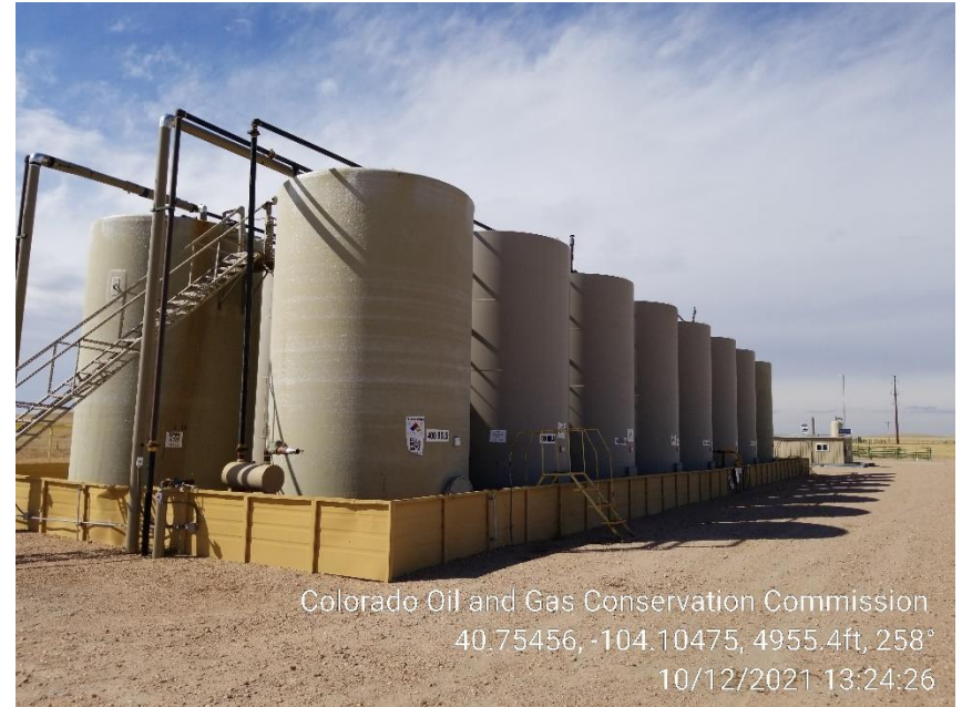
Photo 4 – Tank Battery
