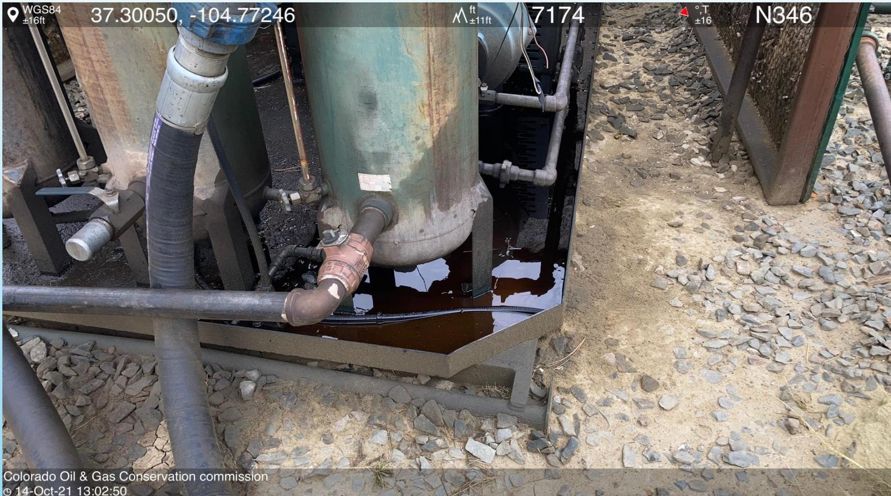
**PHOTO 4: APPEARS TO BE OIL IN COMPRESSOR SKID. COMPLY WITH RULE 1002.f.(2)B, Comply with general provisions of the oil and gas act for wildlife protection AND SB-181. CA DATE 10-15-21.**
