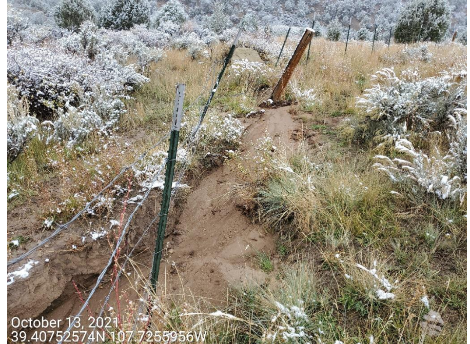
Photo 6: Continued from photo 5. Photos show gully erosion degradation within the ditch due to runoff, as well as sediment transport and deposition.
