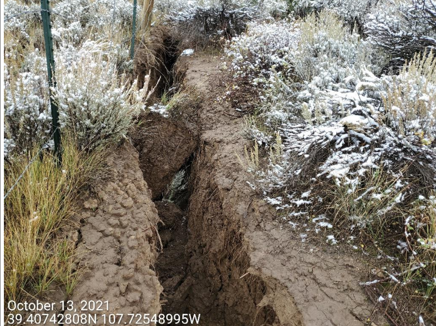
Photo 6: Continued from photo 5. Photos show gully erosion degradation within the ditch due to runoff, as well as sediment transport and deposition.
