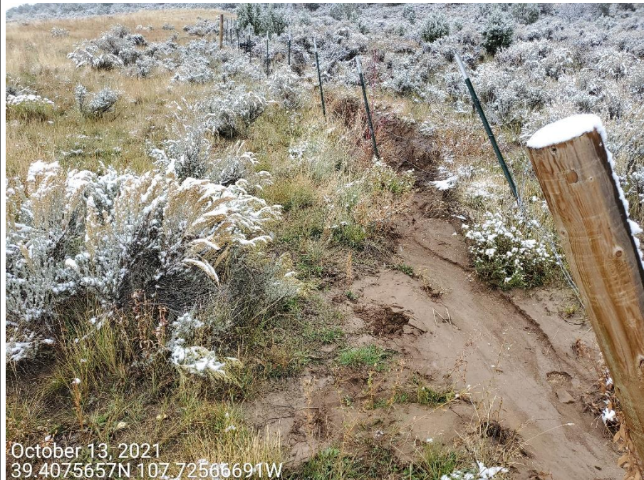
Photo 7: Continued from photo 5. Photos show gully erosion degradation within the ditch due to runoff, as well as sediment transport and deposition.
