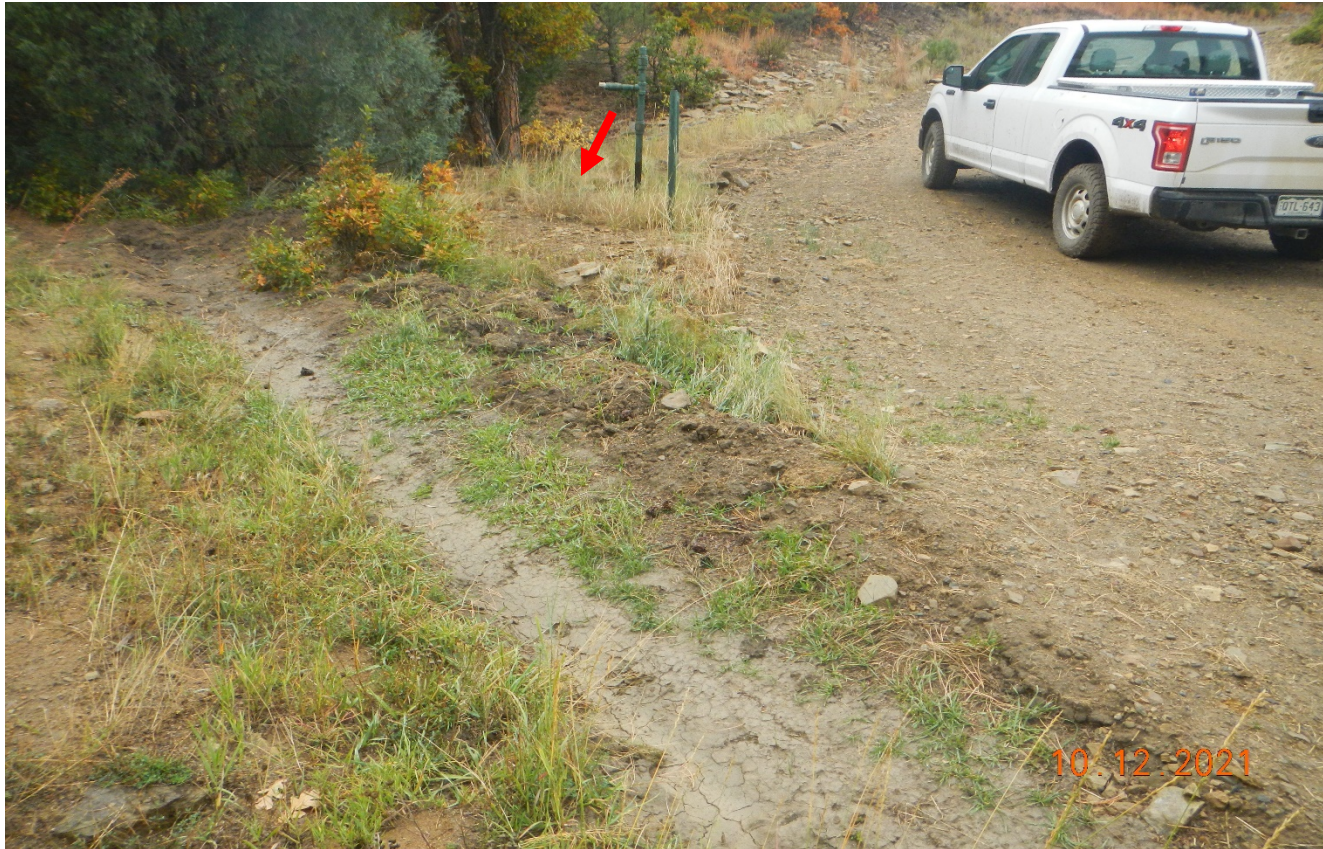
Photo 3. Facing toward the culvert further along the road. Drainage toward the culvert was not corrected. The culvert is shown at the red arrow which to be repaired to allow proper drainage.
