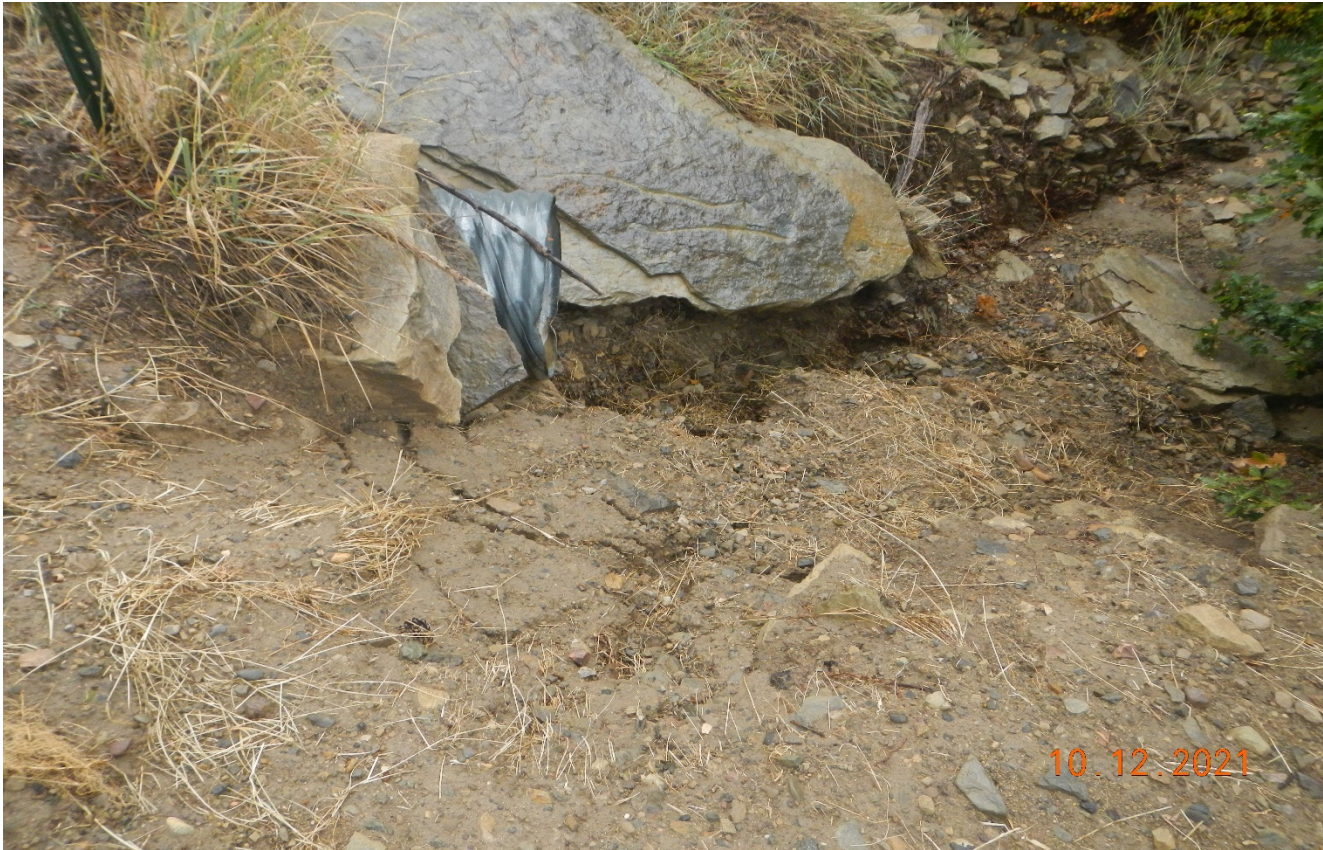
Photo 2. The pipeline has been covered with soil however this is not stabilized. Outlet protection at the culvert is needed.
