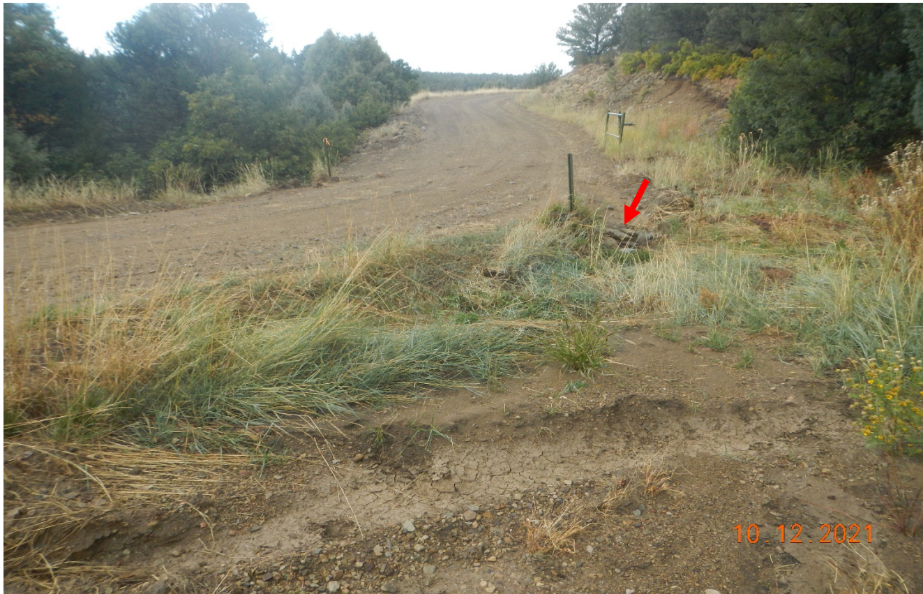
Photo 1. Facing northeast toward the access road. The culvert shown at red arrow is filled in with sediment. Stormwater flowed across the road in this area. The culvert will need to be repaired and proper drainage to the culvert needs to be repaired.
