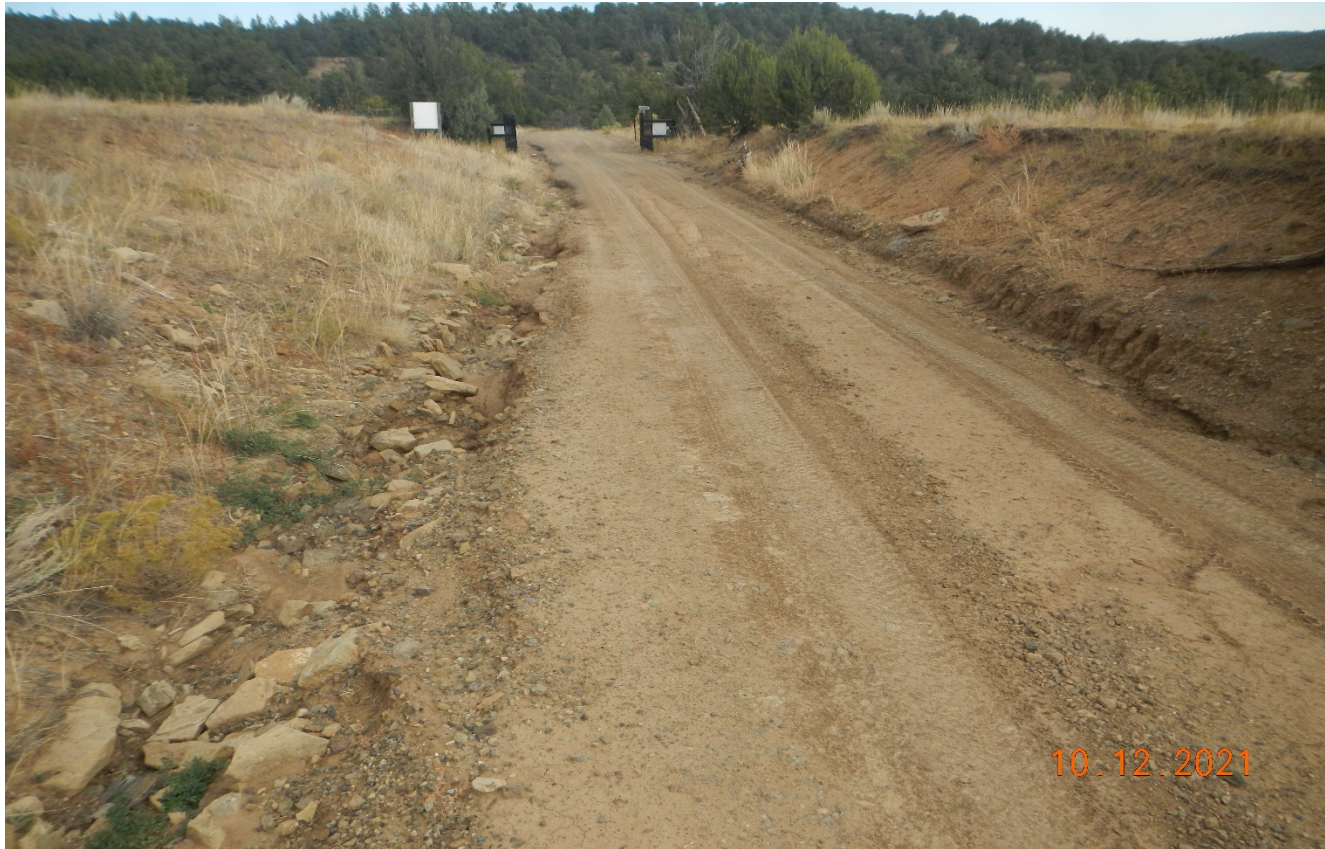
Photo 1. Facing northeast along the main road near the electric gate. Stormwater is directed down the road side in this area which is contributing to erosion further down the county road.
