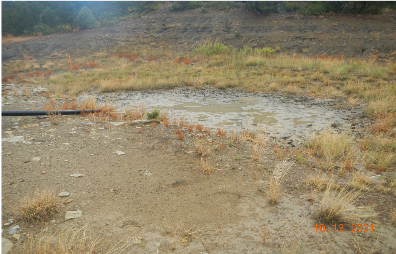
Photo 8. Facing toward the pit. Water level has been lowered. The pit is shallow >2 ft. deep and needs to be constructed to allow 2 ft. freeboard. Earthen berms should be installed around the pit for containment.
