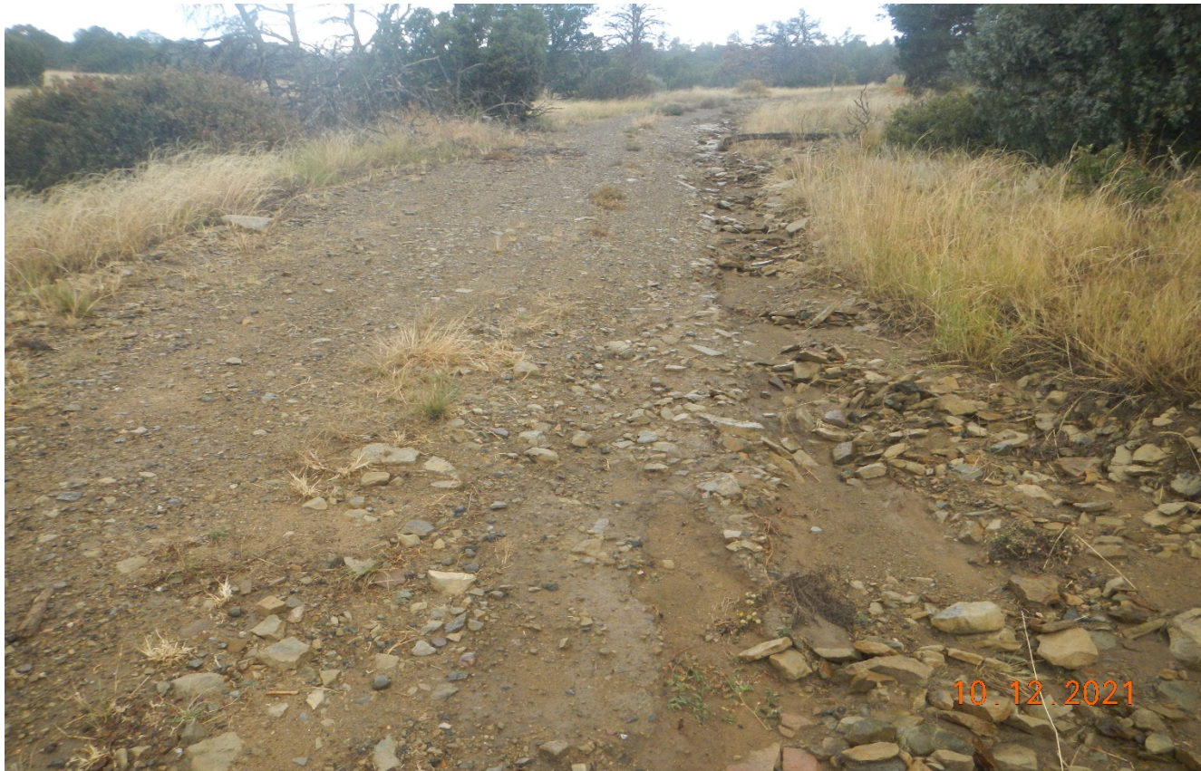
Photo 5. Further west along the access road there is erosion along the road. BMP's need to be installed along the road.
