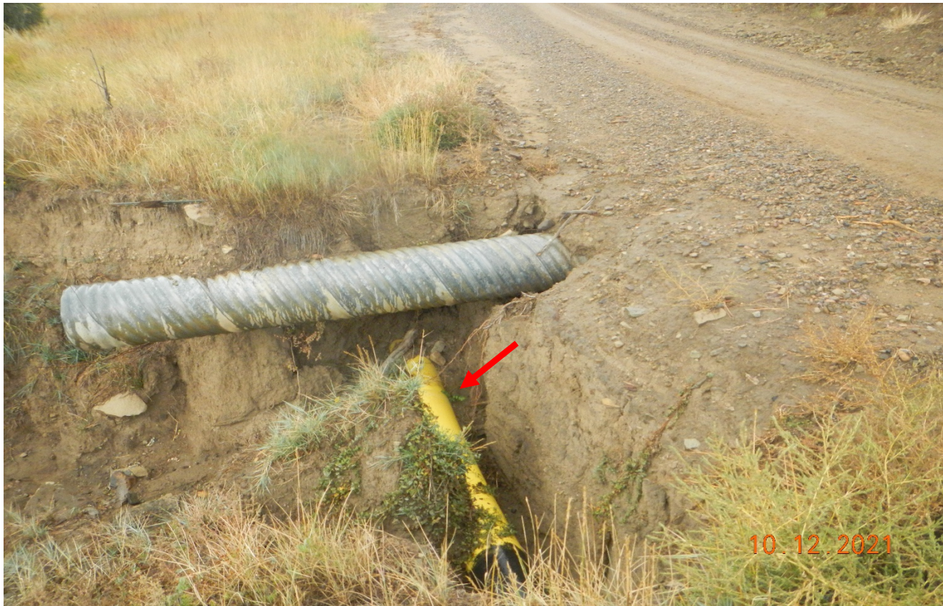
Photo 2. This culvert along the main road is partially washed out and needs to be repaired. There is an exposed pipeline shown at red arrow.
