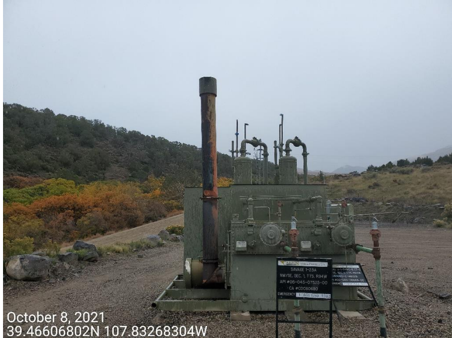
Photo 3: Photo shows bird protection screen is missing from the separator equipment.
