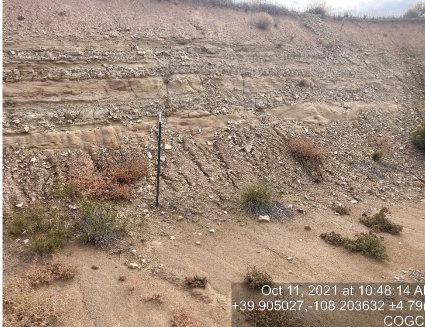
Lack of stabilization/erosion
