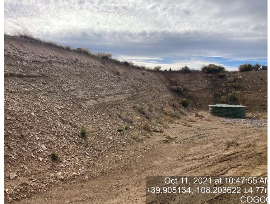
Lack of stabilization/erosion
