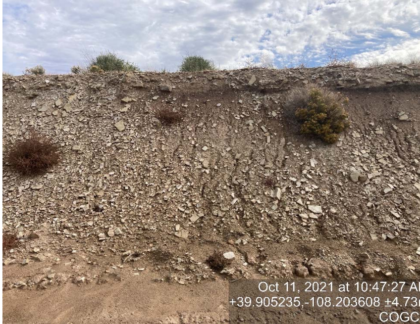
Lack of stabilization/erosion
