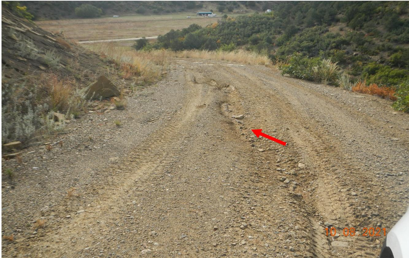
**Photo 6.** Stormwater erosion is occurring down the road shown at red arrow.
