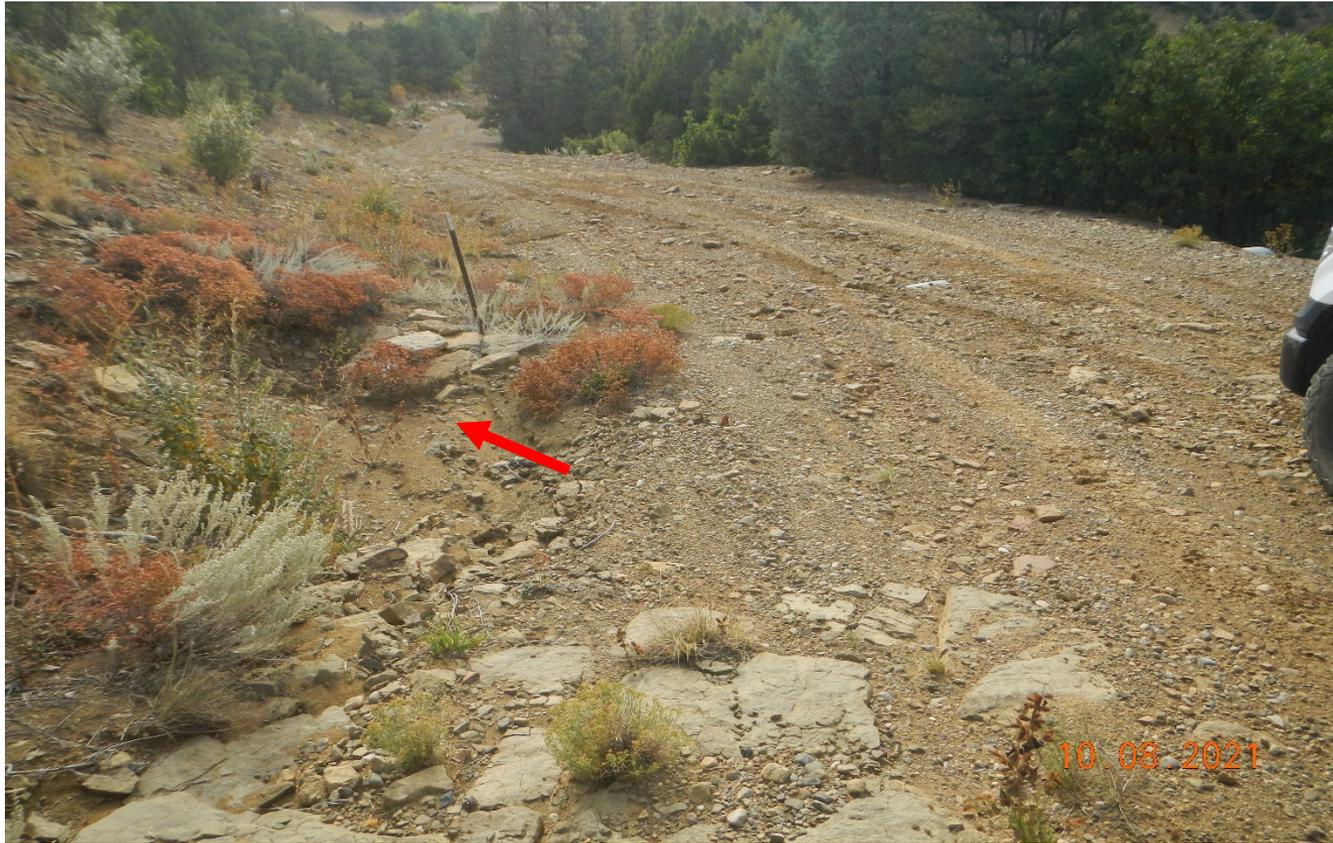
**Photo 7.** There are multiple culverts further along the road that are filled in with sediment that need maintenance.
