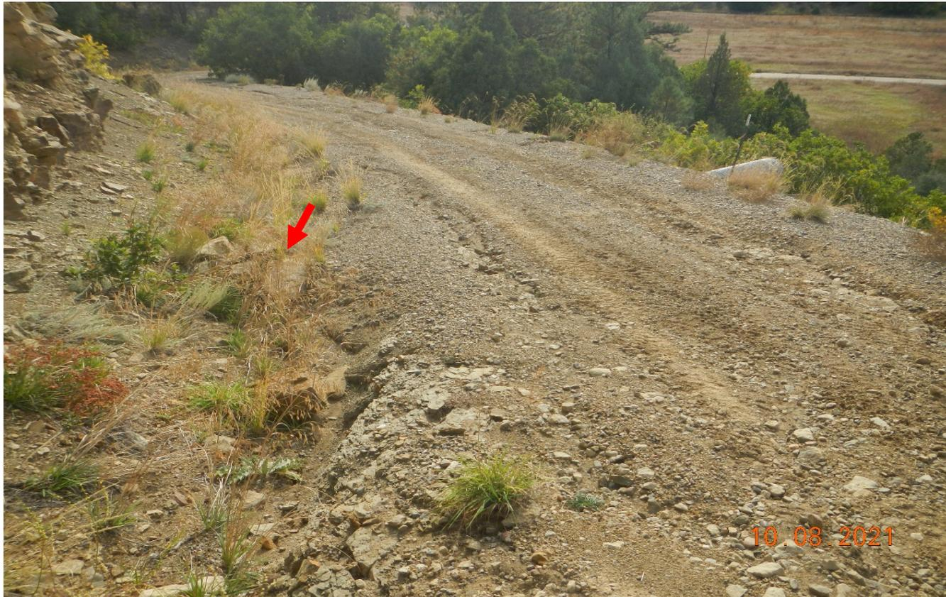
**Photo 5.** Facing southwest further uphill along the access road. There are erosion issues along the road and the culvert show at red arrow is filled in with sediment.
