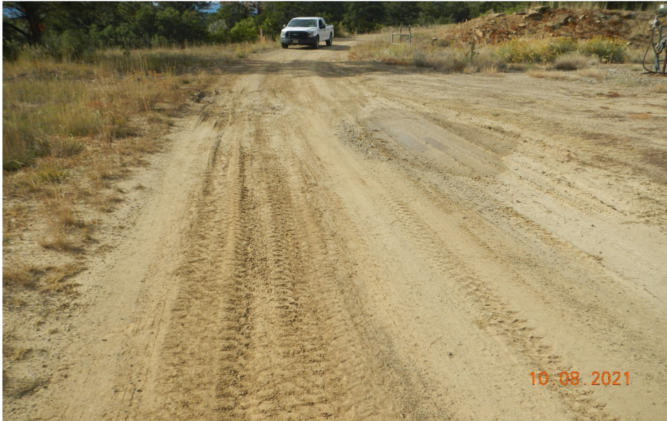
**Photo 10.** Facing northwest at the well site. Stormwater is not properly diverted in this area of the road causing water pooling on the road.
