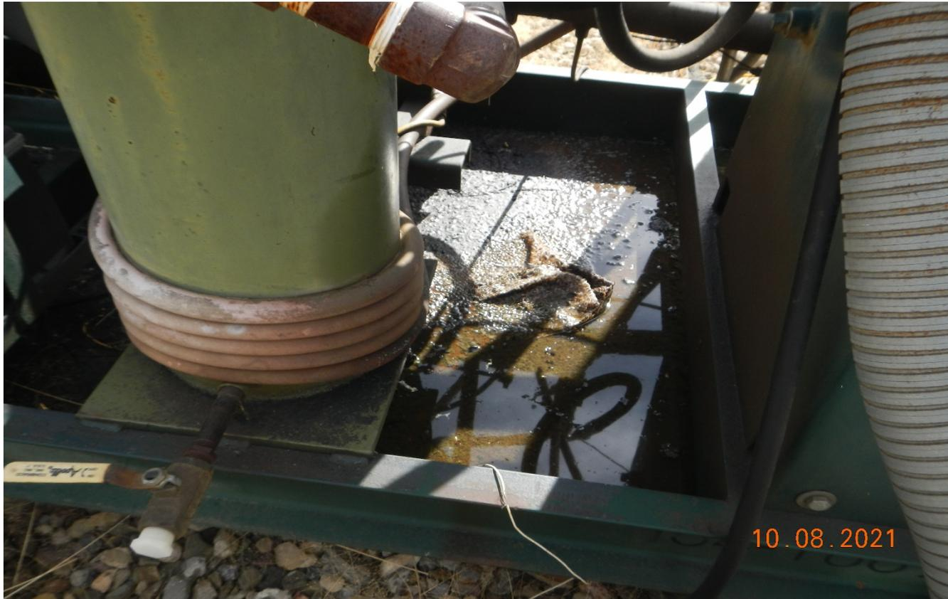
**Photo 14.** There is oily rags found in the engine skid.
