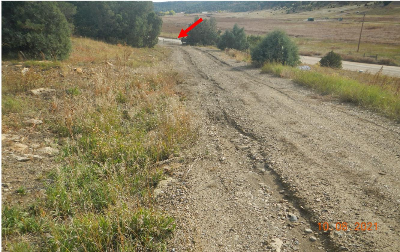
**Photo 1.** Facing south at the access road near the county road, red arrow points to the access gate. There is vehicle rutting in this area.
