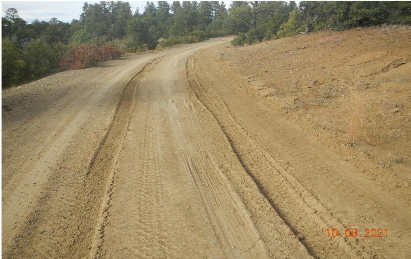
**Photo 9.** Facing north along the access road. There is vehicle rutting occurring in this area and stormwater is not be properly diverted.
