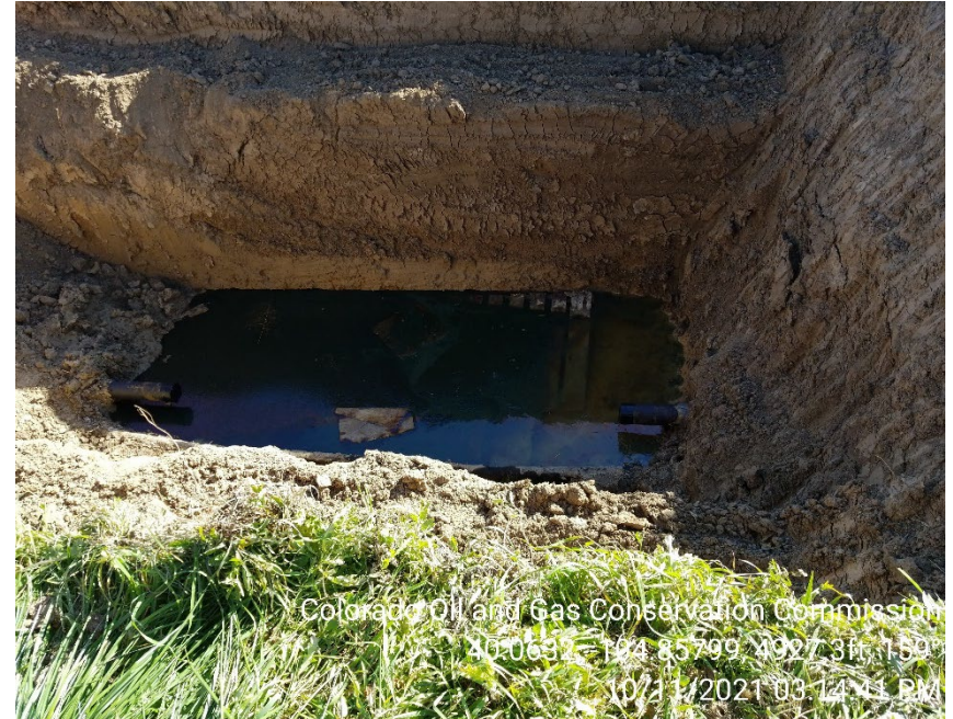
Photo 2 – Spill excavation. Free product observed on groundwater.
