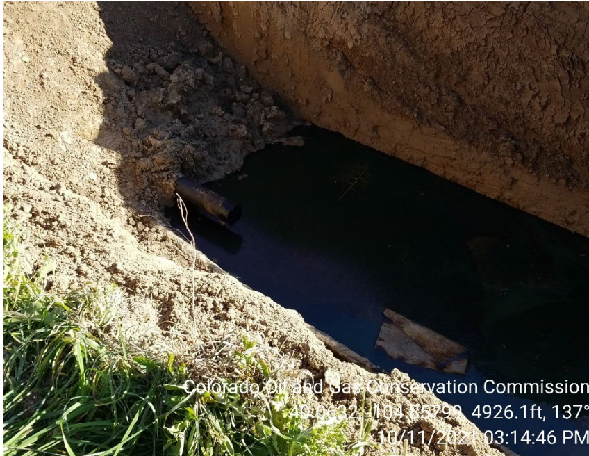
Photo 3 – Spill excavation. Tape placed over cut end of flowline.
