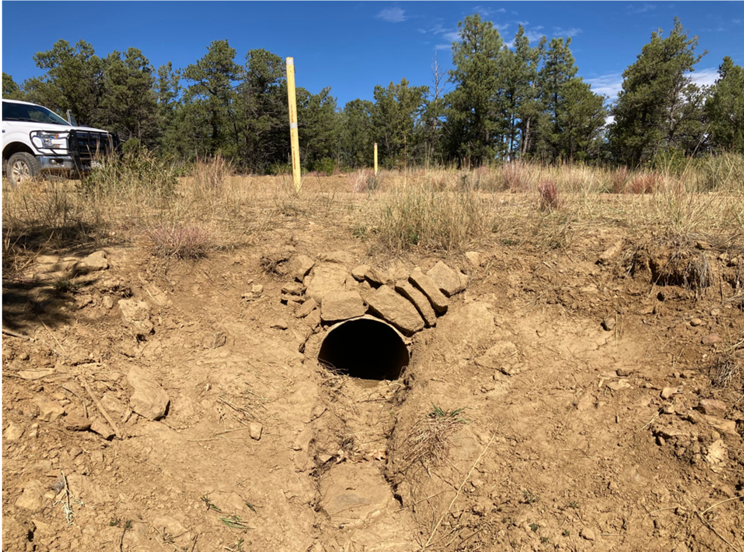
PHOTO 7: THE SEDIMENT ACCUMULATION WAS REMOVED FROM THE CULVERT OUTLET.
