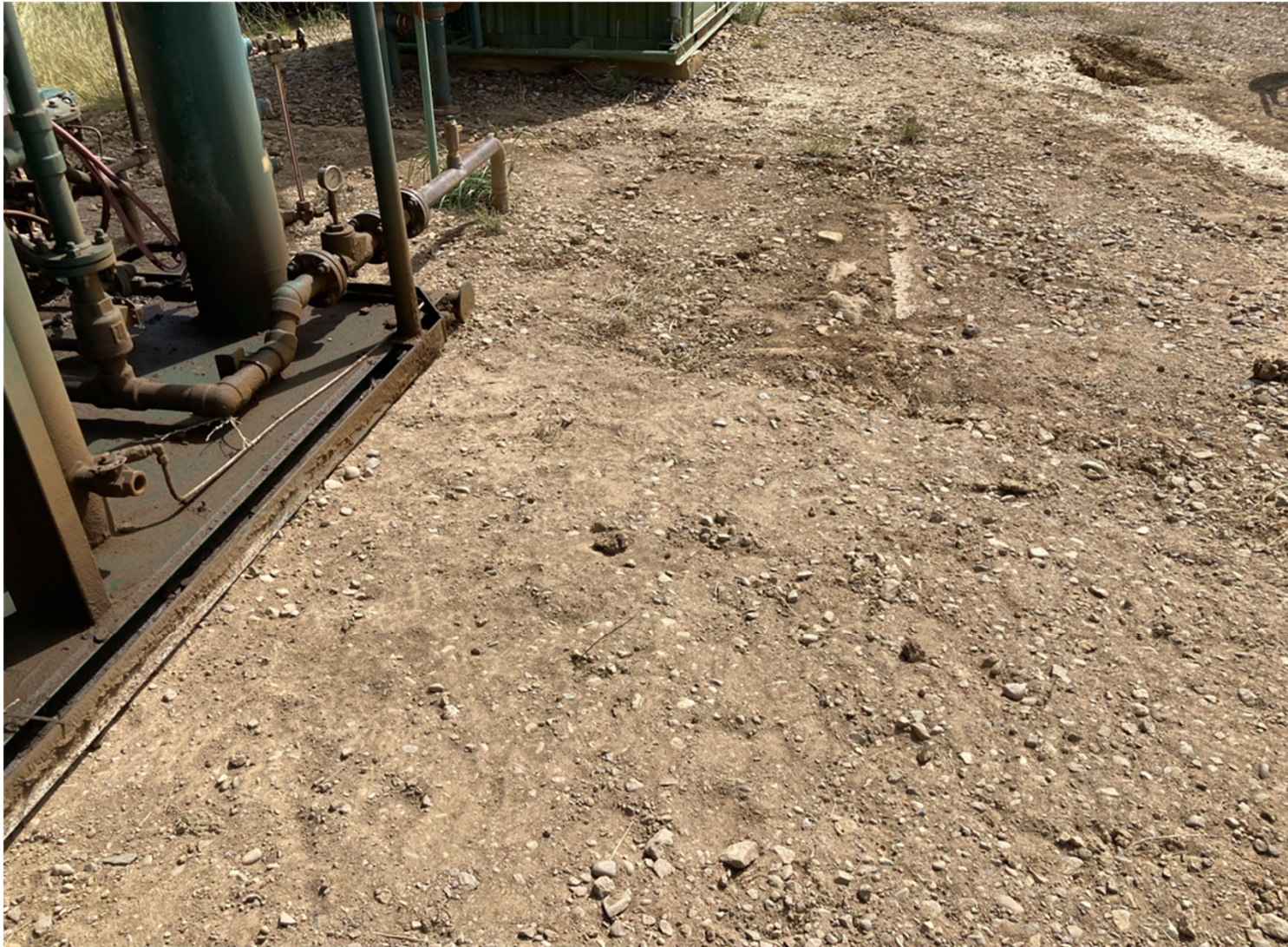
PHOTO 5: THE IMPACTED SOIL NEXT TO THE LIQUID RING COMPRESSOR THAT OVERFLOWED CONTAINMENT WAS REMOVED AND PROPERLY DISPOSED IN ACCORDANCE WITH THE OGRIS OPERATING WASTE MANAGEMENT PLAN. THE COMPRESSOR WAS PLACED BACK TO ITS ORIGINAL POSITION ON THE WELL PAD.
