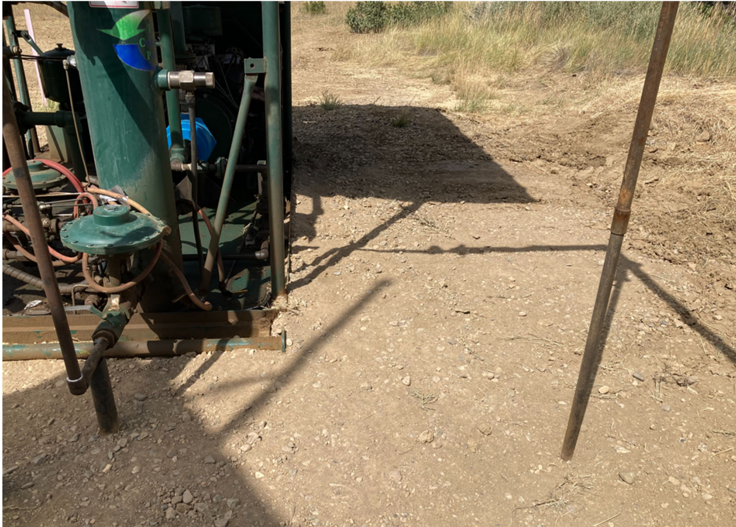
PHOTO 5: THE IMPACTED SOIL NEXT TO THE LIQUID RING COMPRESSOR THAT OVERFLOWED CONTAINMENT WAS REMOVED AND PROPERLY DISPOSED IN ACCORDANCE WITH THE OGRIS OPERATING WASTE MANAGEMENT PLAN. THE COMPRESSOR WAS PLACED BACK TO ITS ORIGINAL POSITION ON THE WELL PAD.
