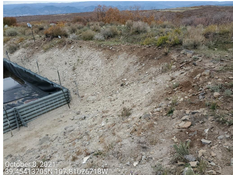
Photo 3: Photos taken from the cut slopes. Photos provide examples showing control measures to protect/stabilize the cut slopes of the location are missing or insufficient.
