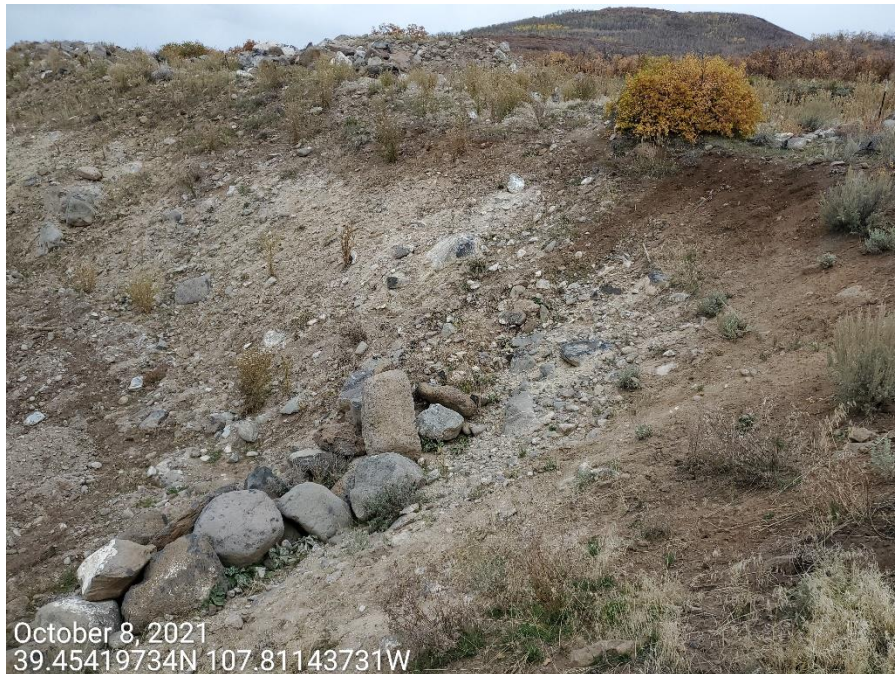
Photo 3: Photos taken from the cut slopes. Photos provide examples showing control measures to protect/stabilize the cut slopes of the location are missing or insufficient.
