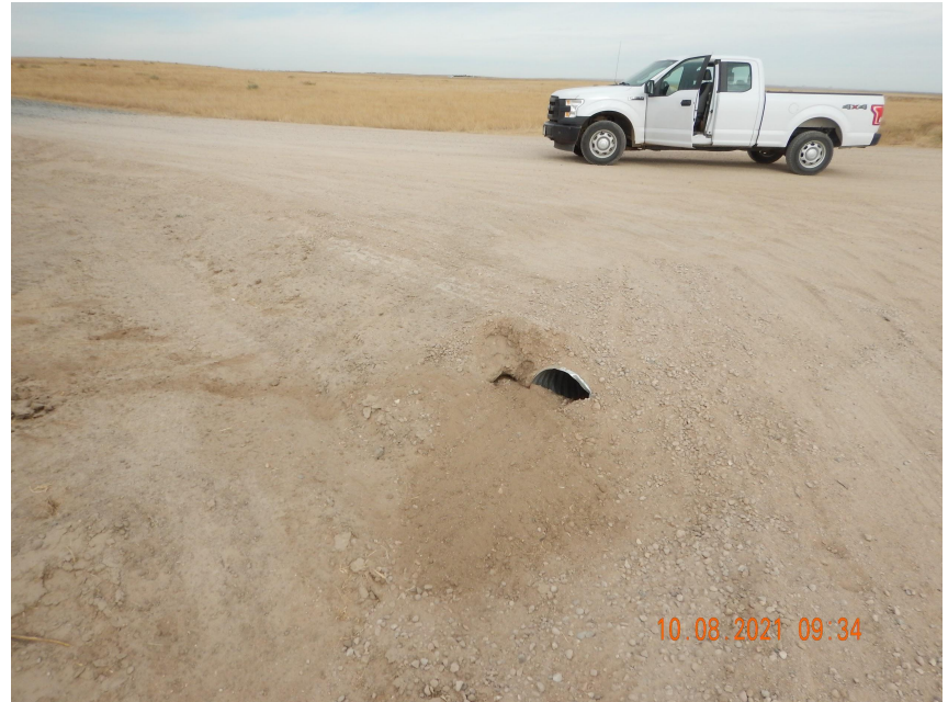
Photo 7. Photo taken from the entrance of location off CR 121, facing North. Photo illustrates culvert needs maintenance, as it is currently blocked with gravel.
