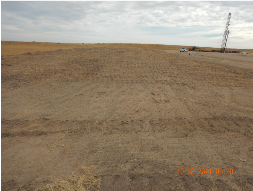
Photo 12. Photo taken from the western topsoil stockpile, facing East. Photo illustrates the stockpile has been temporarily stabilized.
