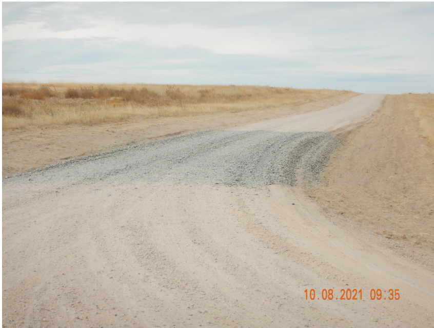
Photo 8. Photo taken from the entrance of location off CR 121, facing West. Photo illustrates a vehicle tracking device BMP.
