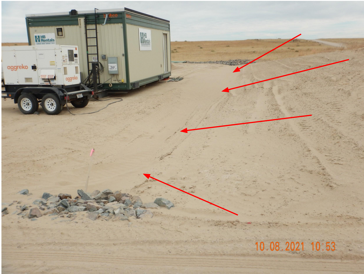
Photo 15. Photo taken of the southeastern ditch BMP, facing East. Photo illustrates sediment accumulation from unconsolidated soil material from the well location due to wind erosion. The well location has not been properly stabilized.
