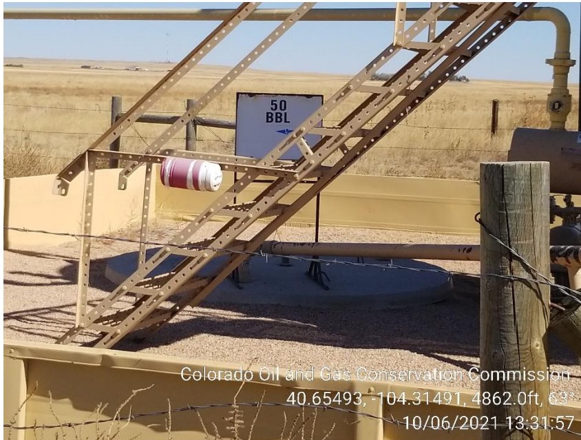
Photo 9 – Missing NPFA and Content Labels
