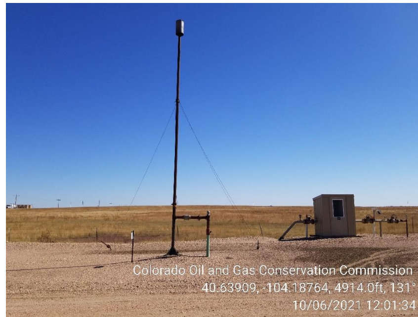
Photo 2 – Flare and Gas Meter – Missing Calibration Card
