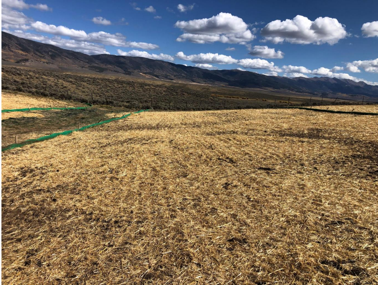
Picture 9: Contour crimping will help with erosion in the draw.
