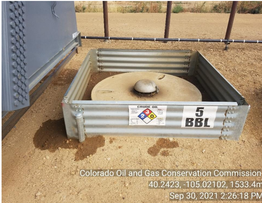
Photo 7 Stained soil in and around Crude oil concrete vault.
