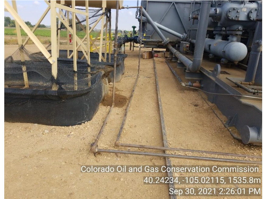
Photo 6 Stained soil under motor oil storage tanks
