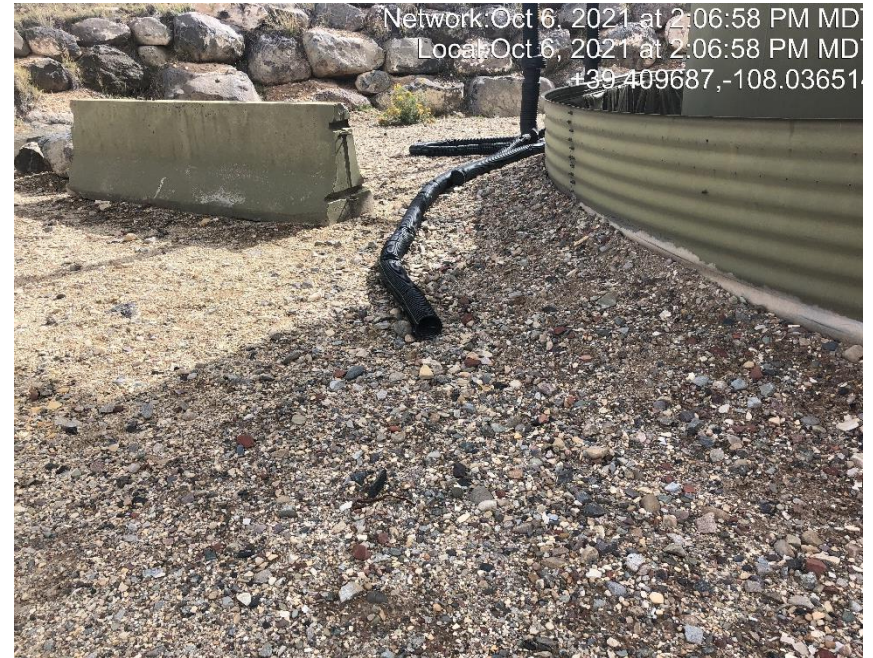
Photo #5026 Flowline heating insulation open ended and not capped.
