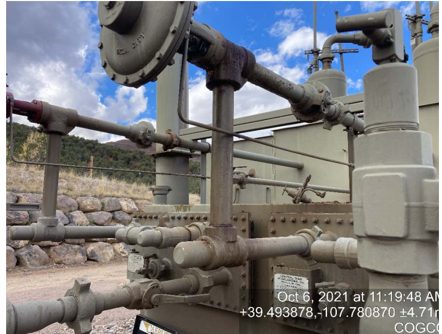
Leaking A-valve or angle body
