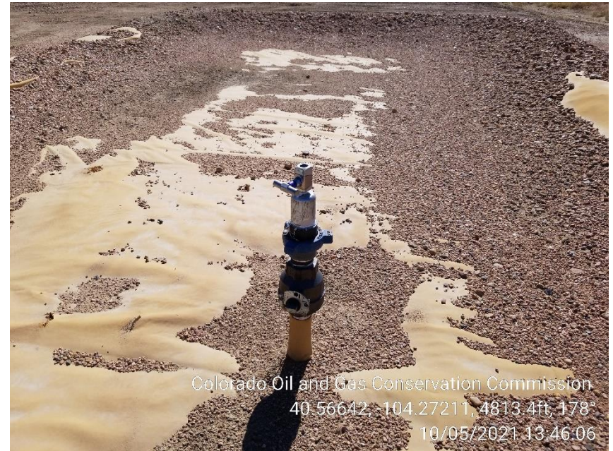
Photo 4 – Unmarked Riser at Gas Meter
