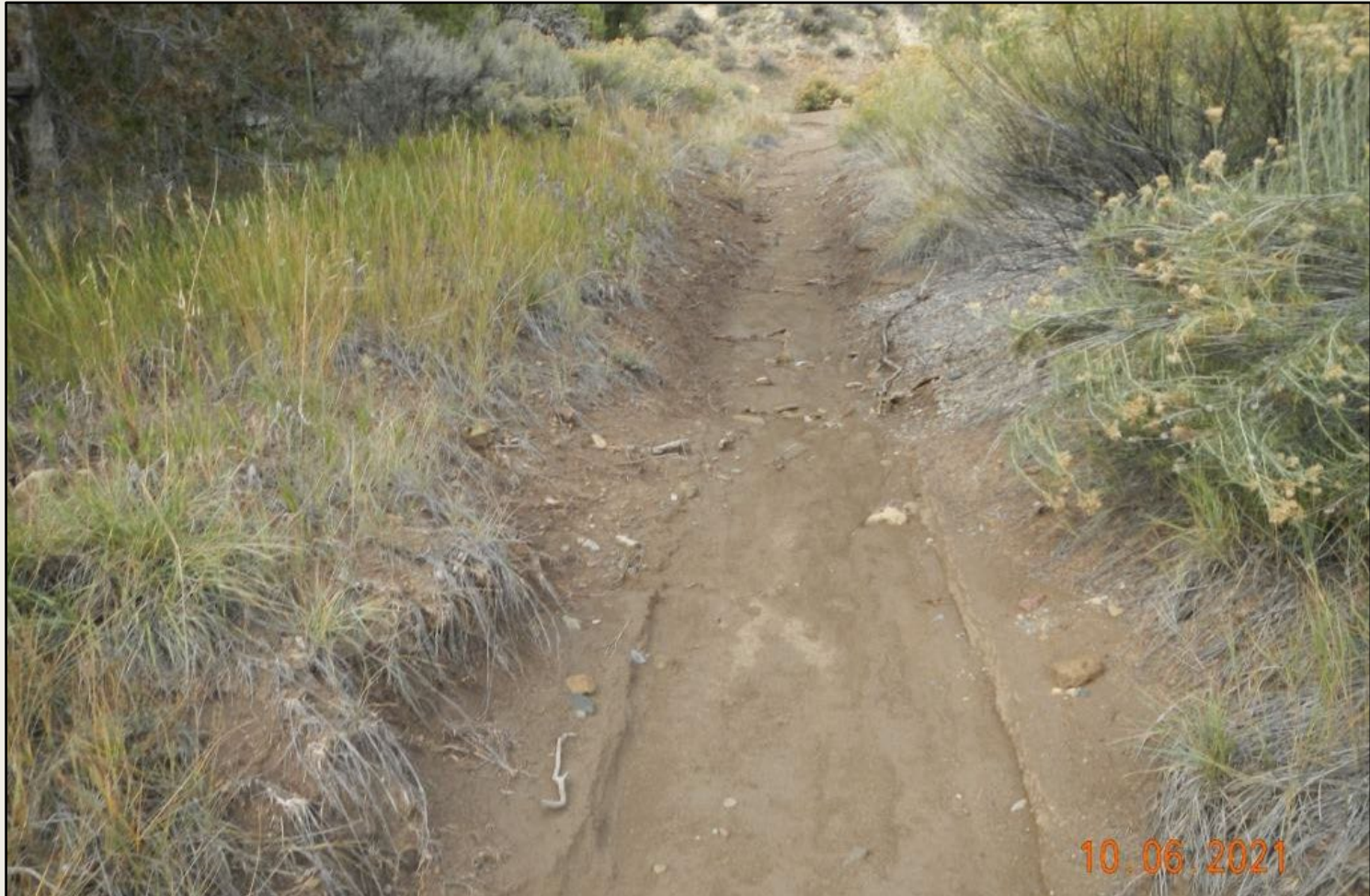
Photo 4. View of southern diversion channel, largely full of sediment and eroding. BMPs need to de-energize channel where velocities are high, and sediment needs to be contained.
