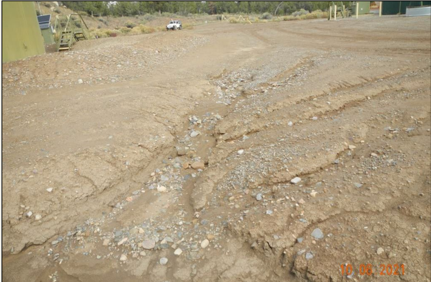
Photo 6. View of area on the southern well pad where stormwater flows off of the well pad toward diversion in photos 4 and 5.
