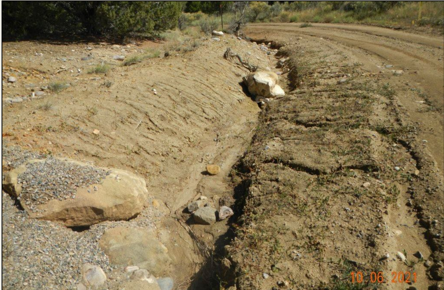
Photo 7. View of erosional channel along the access road. Stabilization is needed on the bed and banks of roadside diversions.
