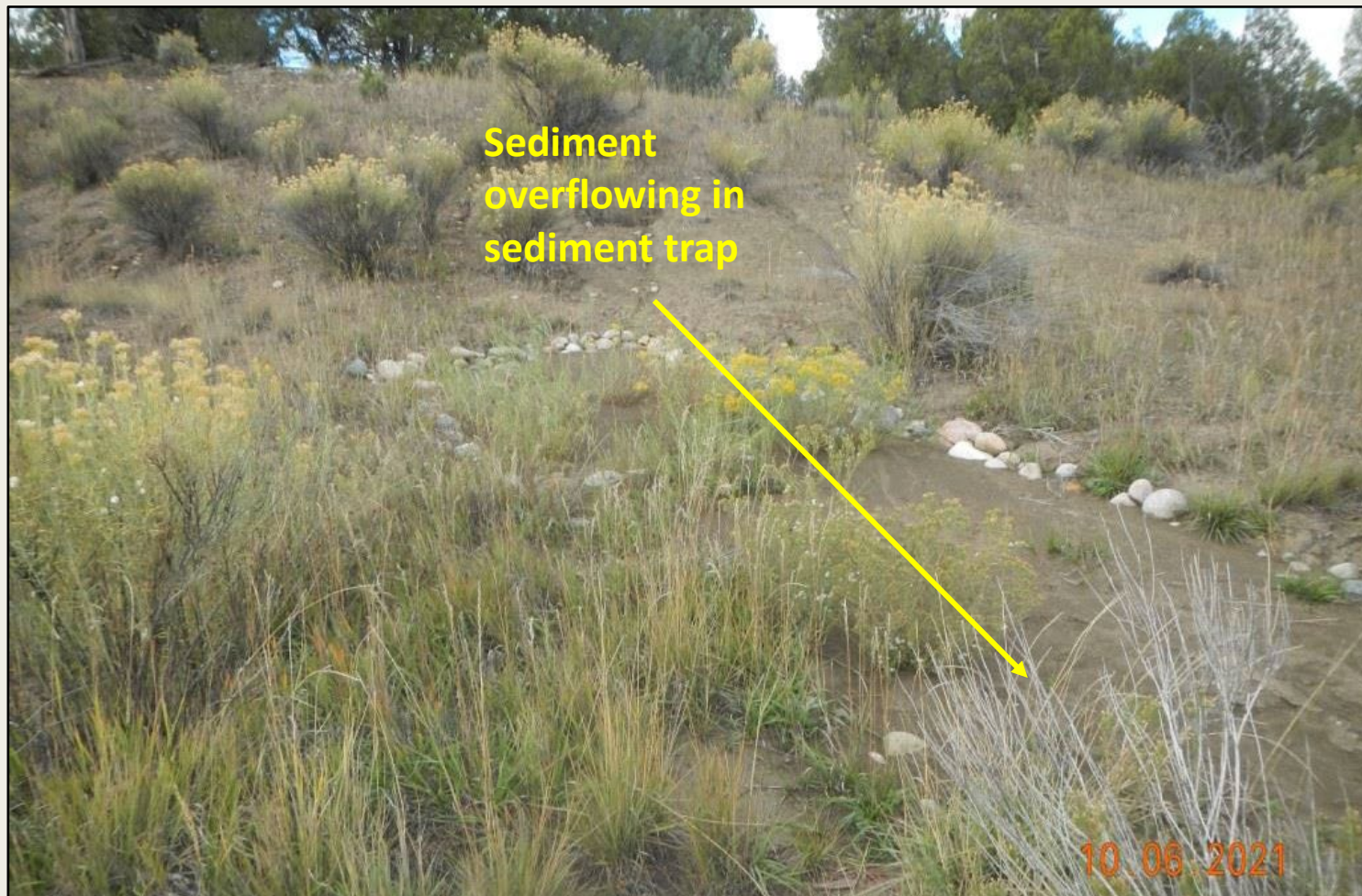
Photo 3. View of silt trap full of sediment in the northwestern project area.
