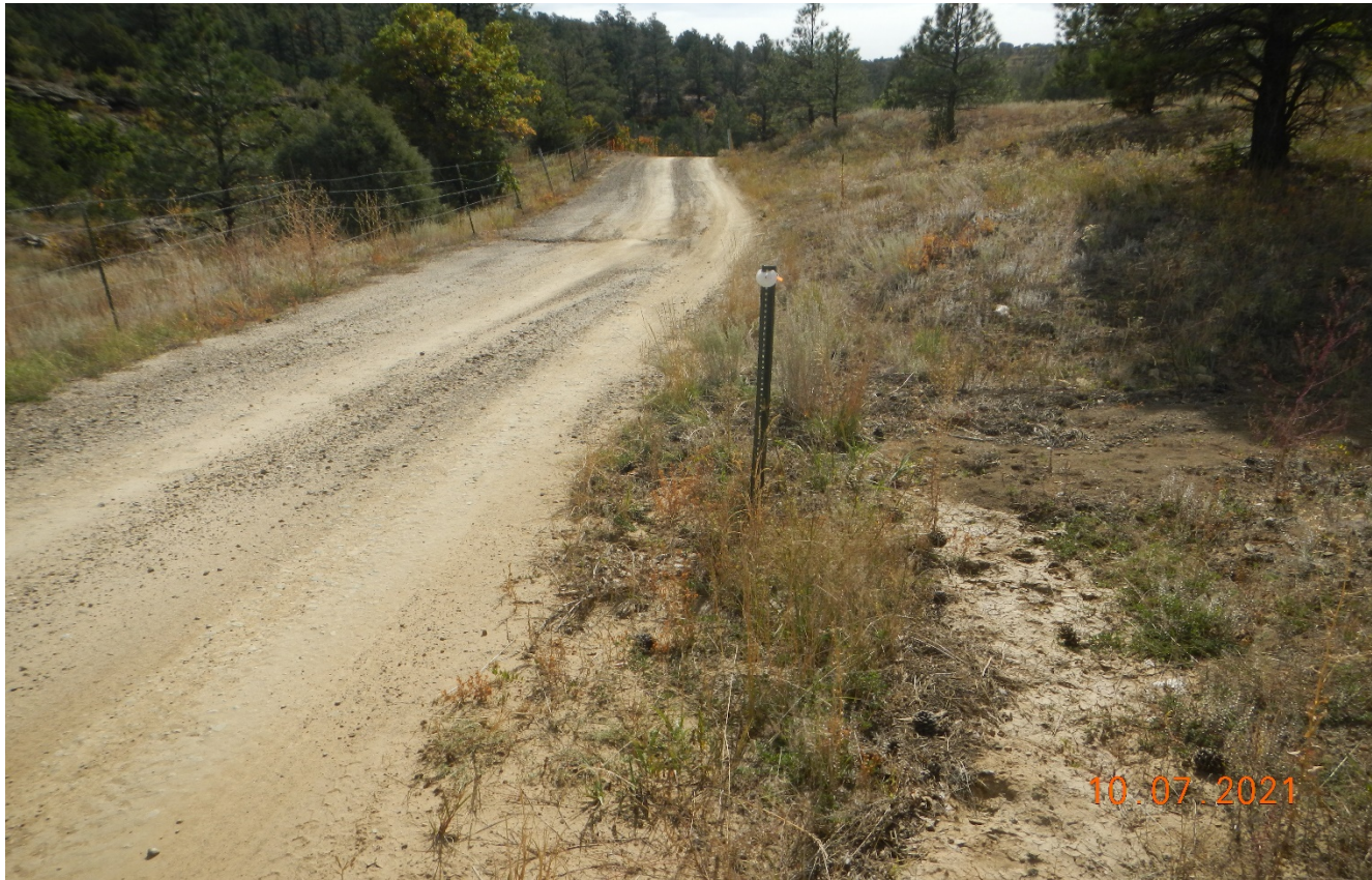
Photo 3. There is a culvert filled in with sediment causing stormwater to flow across the road. Lat/Long:37.16720,-104.82237.
