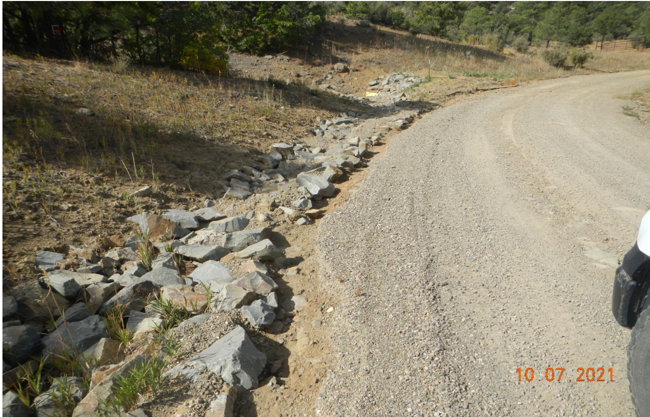
Photo 2. Facing west along the road where BMP's were installed last. Stormwater has eroded around the rock rip rap and needs to be repaired.
