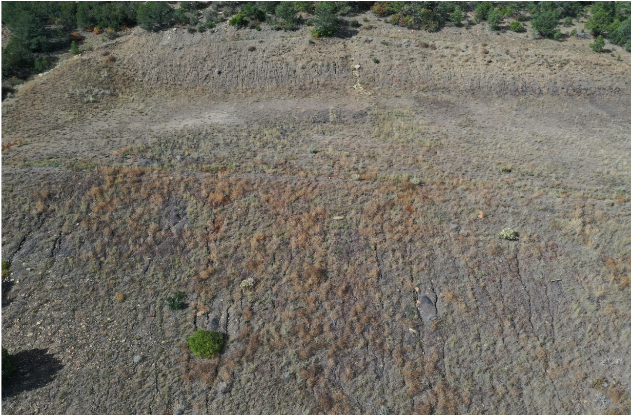
Photo 13. Facing down toward the location shows erosion along the fill slope.
