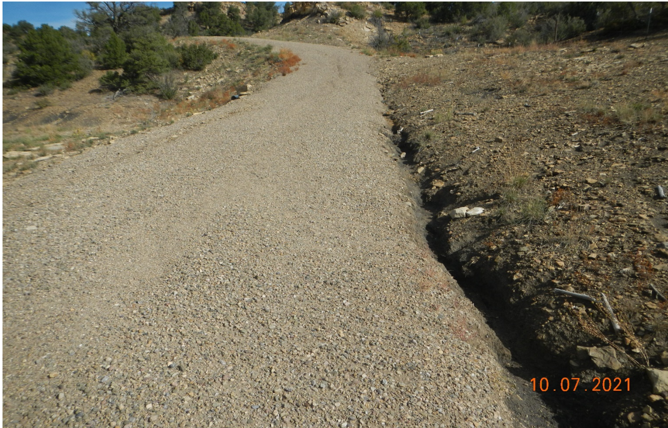
Photo 2. Facing northeast along the access road. The road has not been recontoured and reclaimed. There is an erosion channel developing along the roadside.
