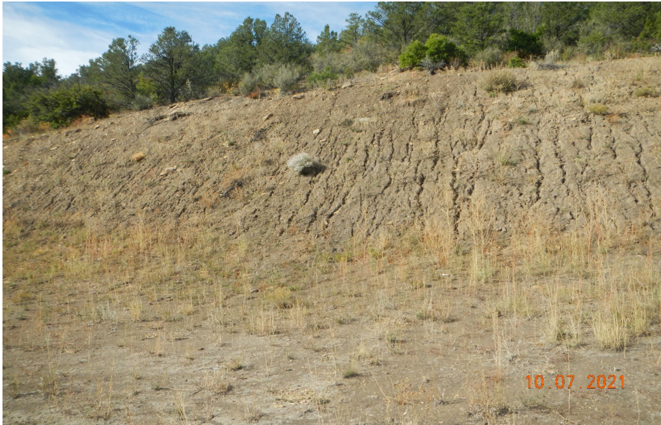
Photo 9. There are signs of erosion occurring off the cut slope.
