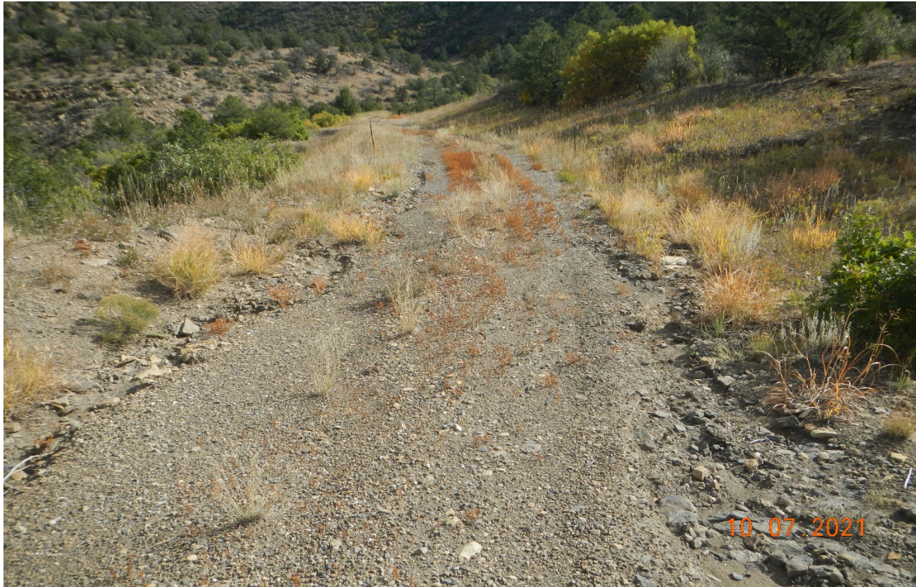
Photo 3. Facing east along the access road. There is erosion along this area of the road.
