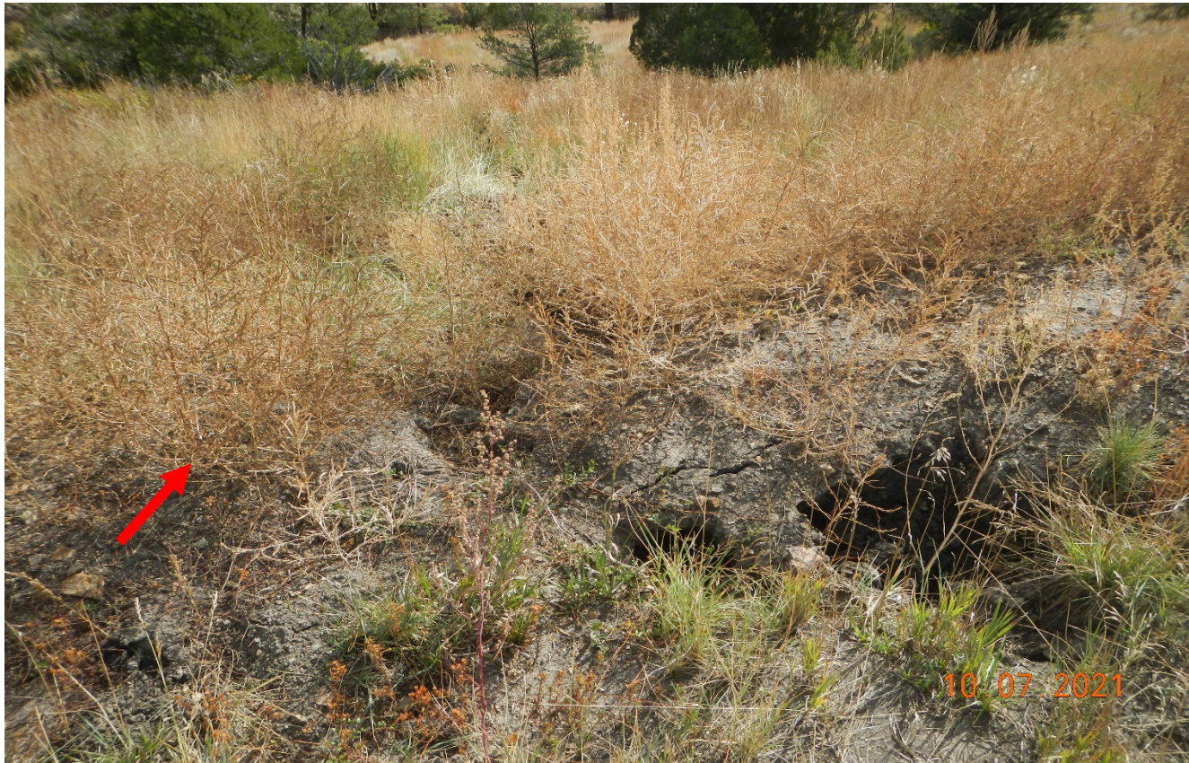
Photo 7. There are erosion channels along the fill slope which can be seen better in aerial imagery (photo 13). Arrow points to undesirable weeds, Russian thistle.
