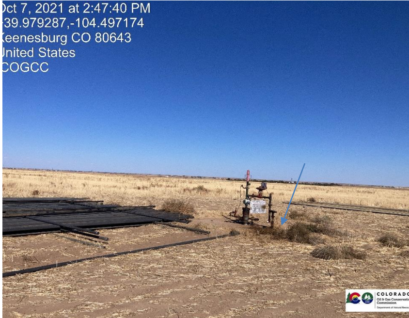
Pic 1 wellhead, tubing and stained soil by wellhead.
