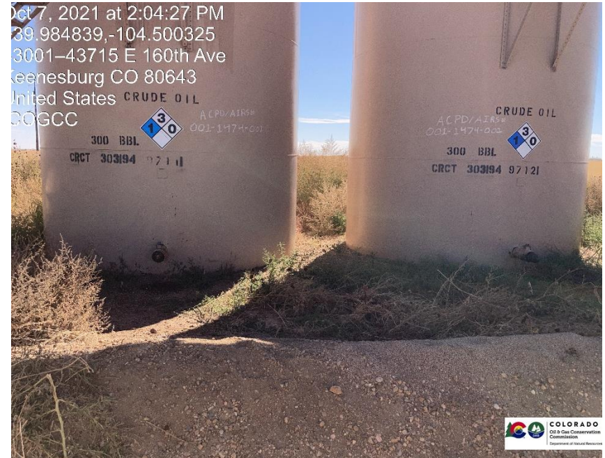
Pic 4 tanks, stained soil under load lines on tanks
