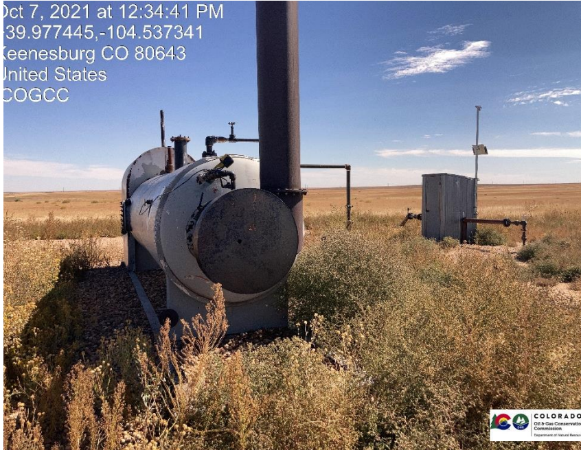
Pic 5 Separator, and gas meter run, weeds unmanaged on location
