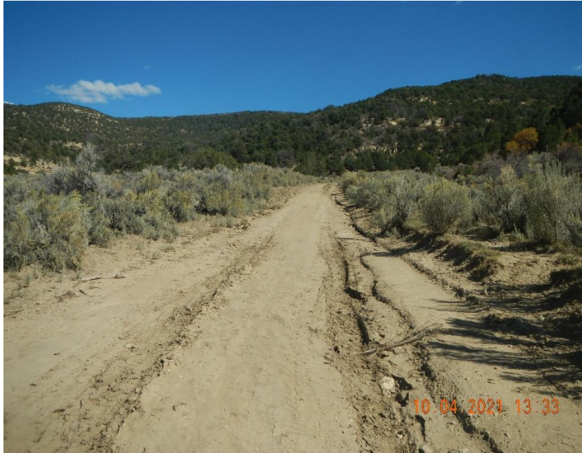
Sediment movement on access road. Washing and rilling of road surface and ditches.
