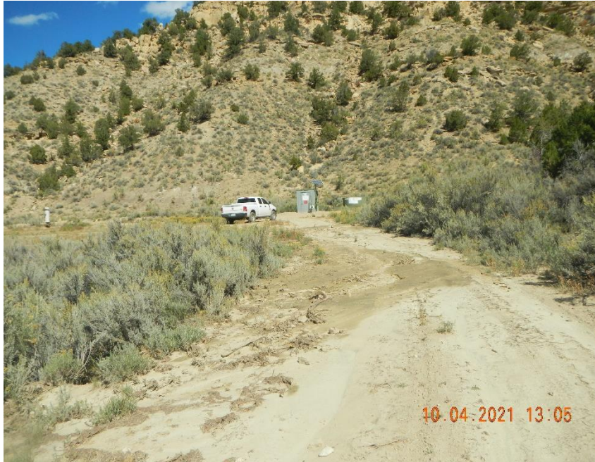
Sediment moving onto roadway at entrance.
