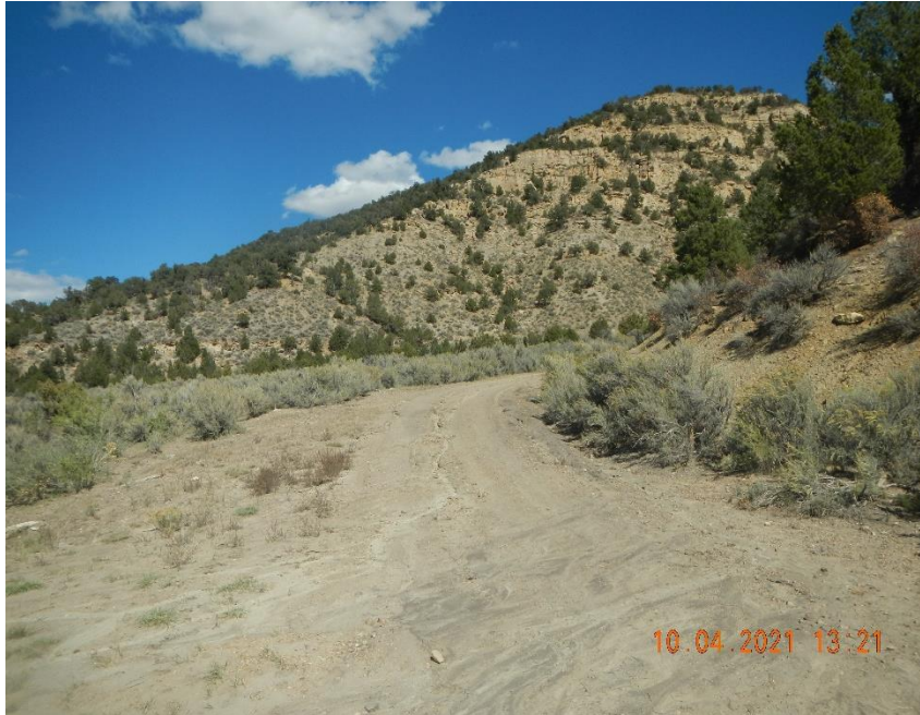
Washing and sediment movement on access road.
