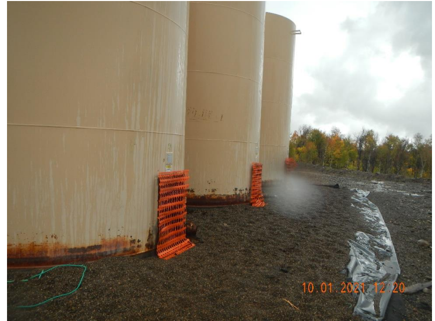
Tank access for heat element has been covered with plastic orange fencing.
