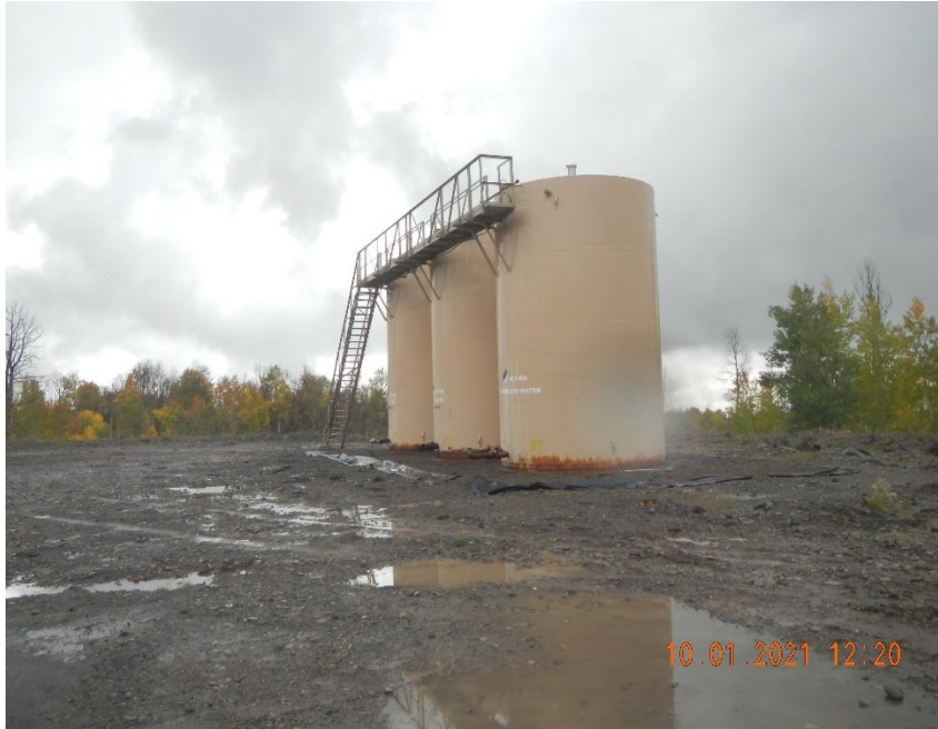
Unused tanks. Metal berm taken down.
