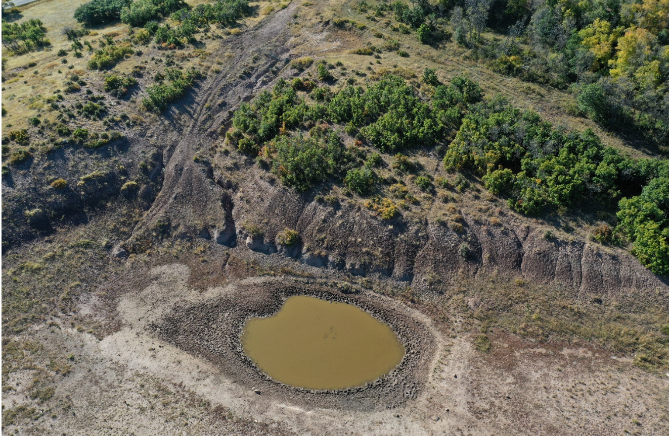
Photo 6. The pit remains and is filled in with stormwater. This photo shows the erosion along the cut slope.
