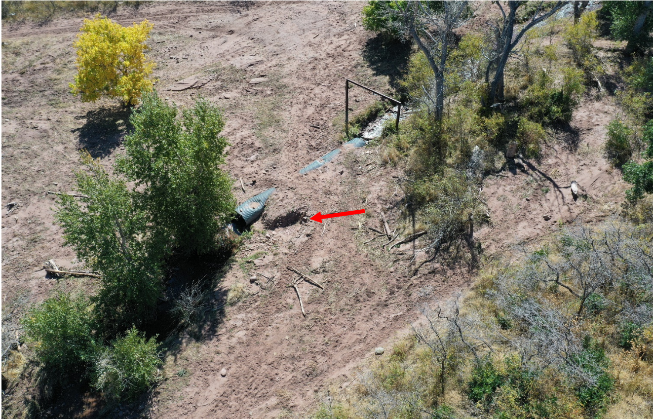
Photo 3. Facing down toward the stream crossing which has eroded around the culvert and may become washed out with the next storm event or snow melt runoff.
