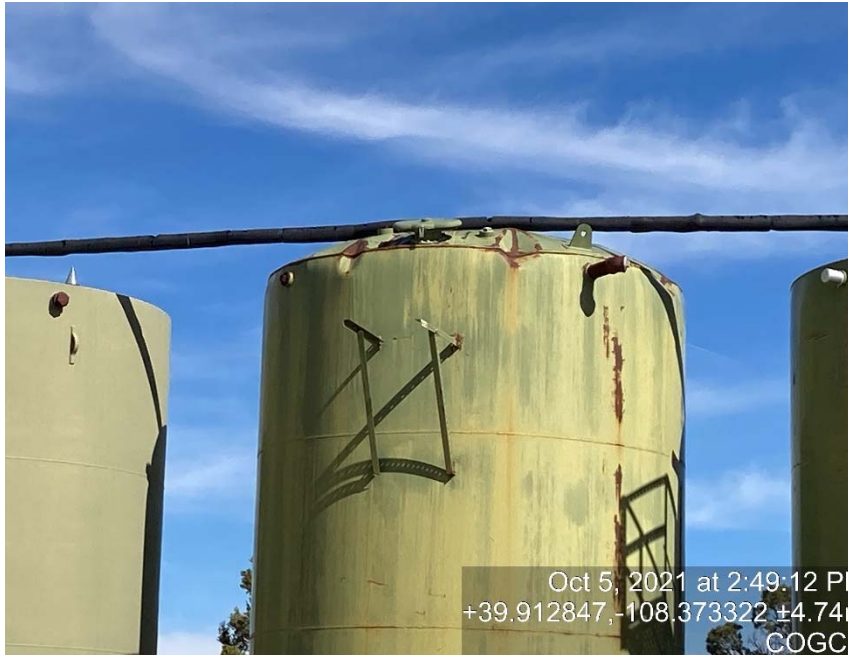
Tank appears to have been over pressured
