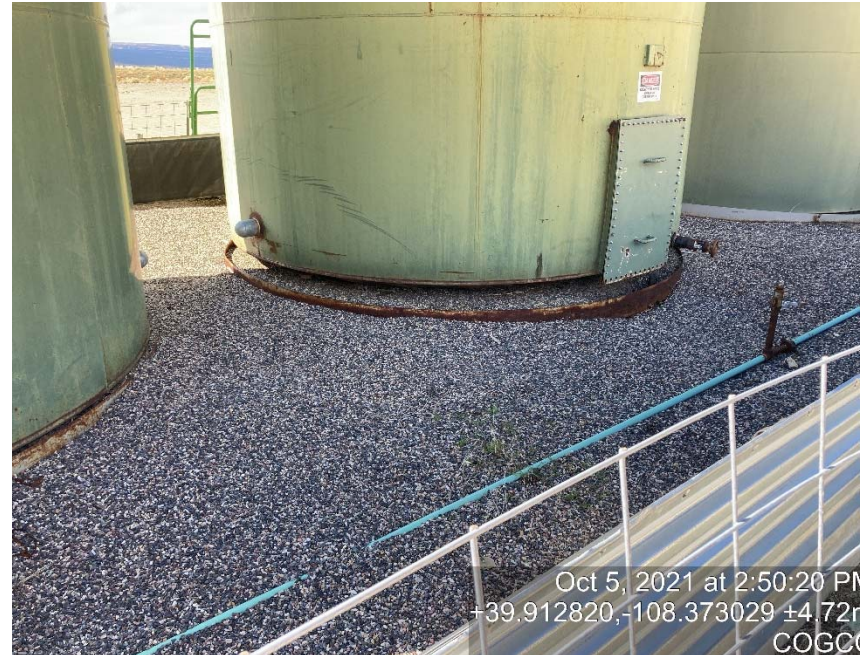
Tank appears to have been over pressured
