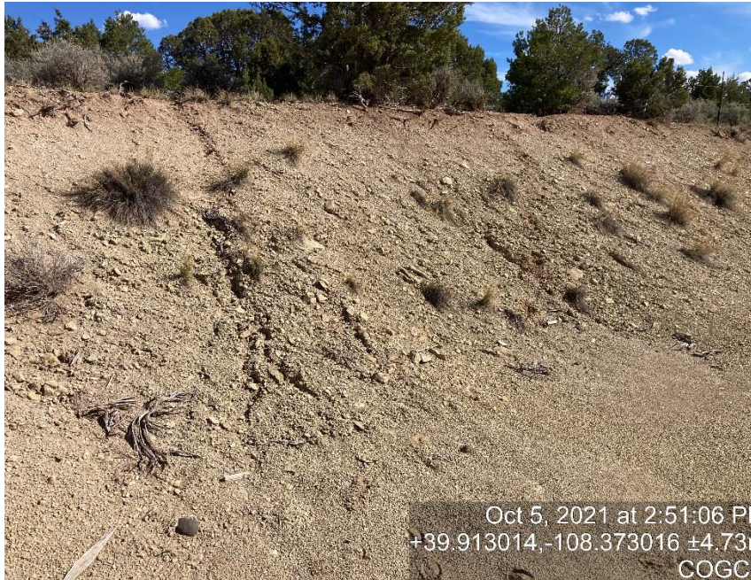
Lack of stabilization/erosion
