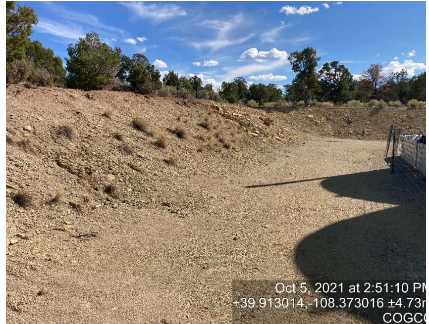
Lack of stabilization/erosion
