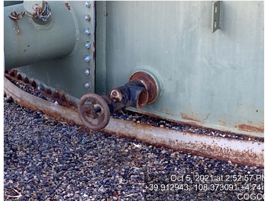
Missing bull plug/cap
