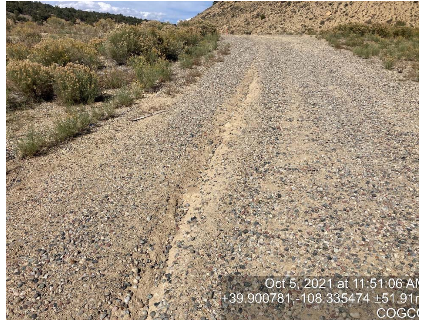
Erosion on access road
