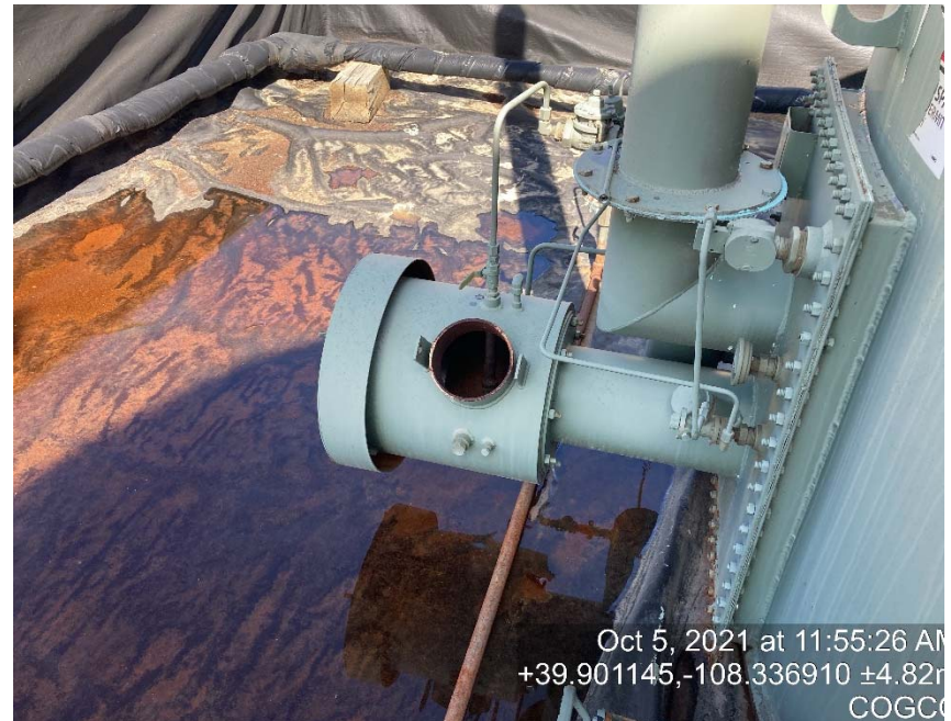
Tank burner missing cap/access for wildlife
