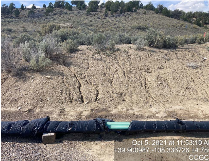
Lack of stabilization/erosion
