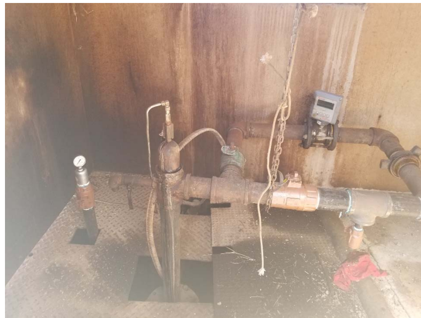
Photo 2. Bradenhead access has been installed.
