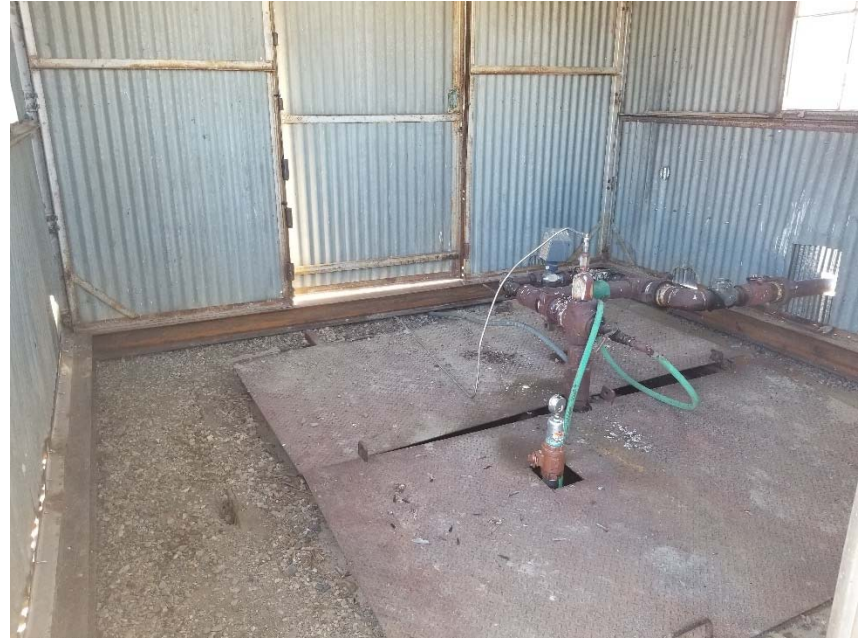
Photo 2. Bradenhead access has been installed.
