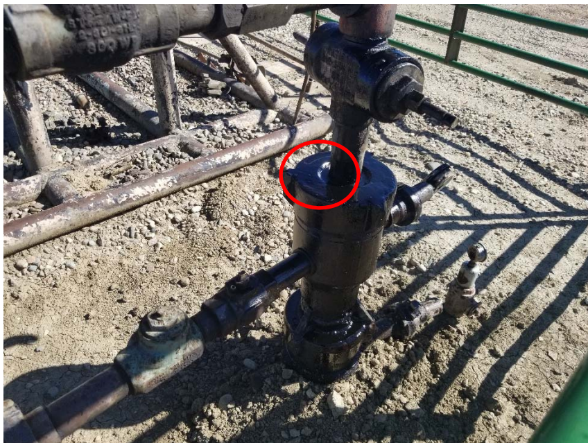
Photo 2. Leak occurring at wellhead.
