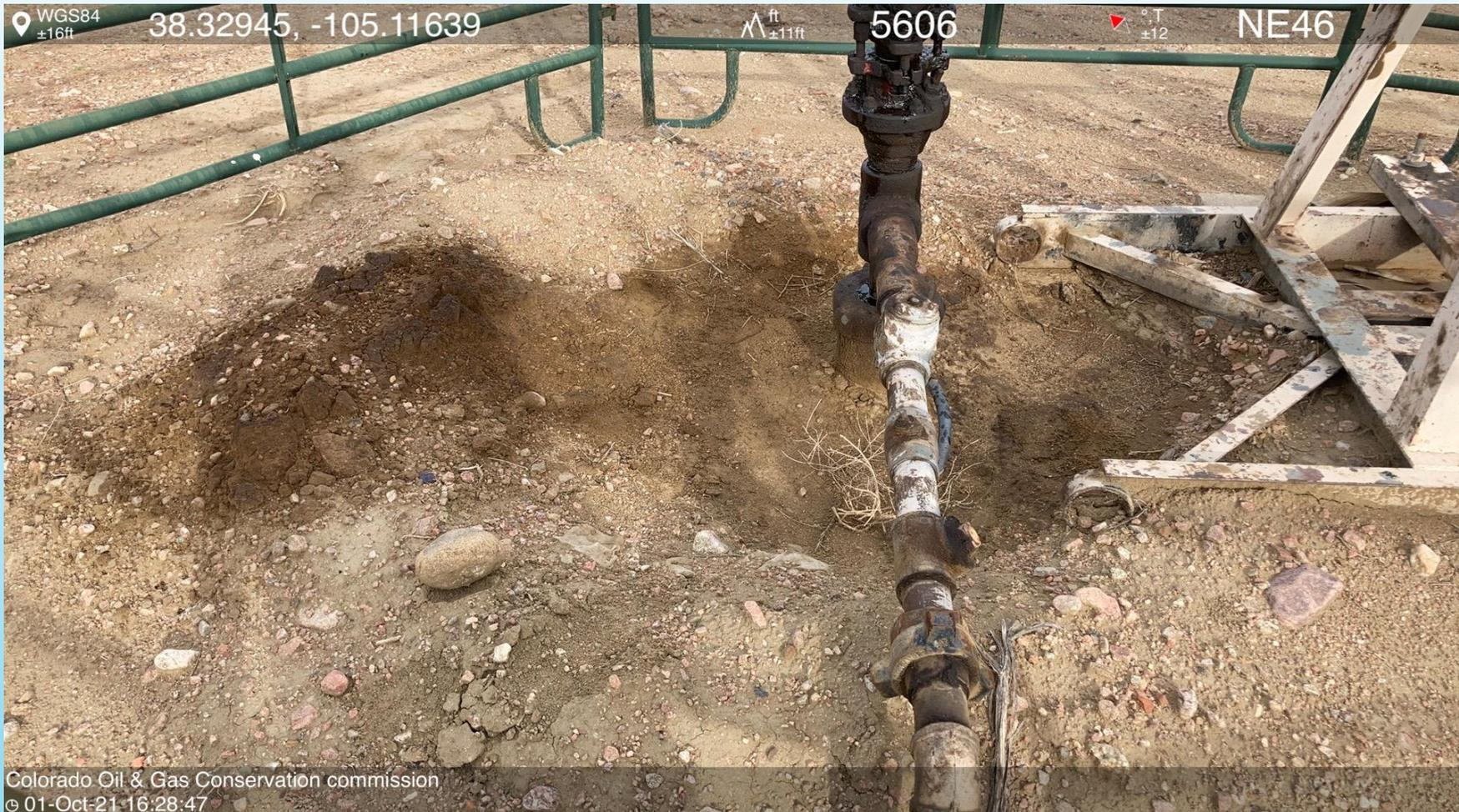
**PHOTO 4: AREA OF IMPACTED SOIL APPEARS TO BE CUDE OIL STAINING FROM LEAKING WELLHEAD. Conduct maintenance on equipment, cleanup stained material and review self inspection processes. (FIX LEAKING WELLHEAD). COMPLY WITH RULE 1002,.(2).D CA DATE 10-8-2021.**
